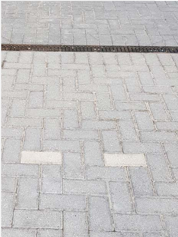
Block paving to customer walkways
