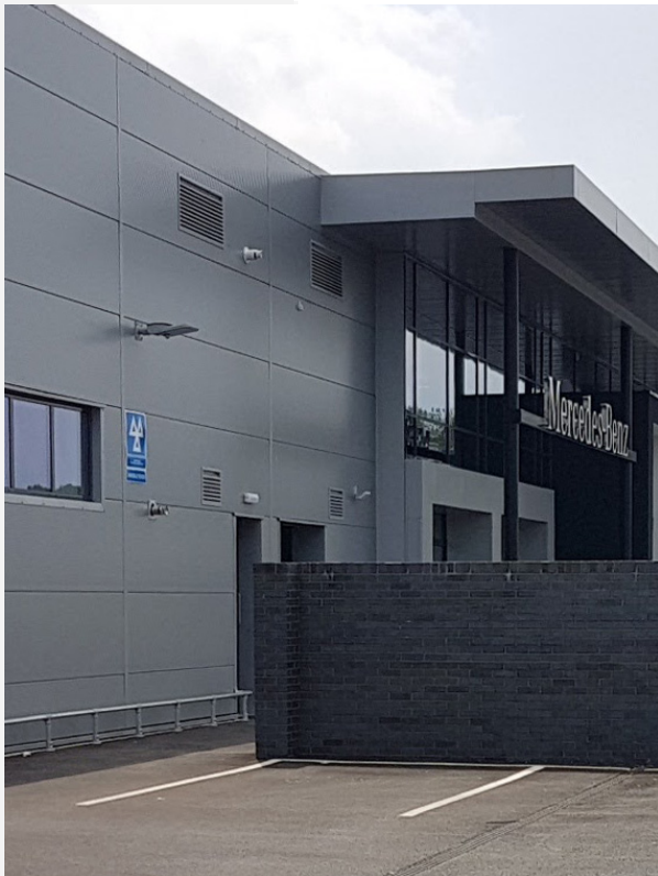
Back of house cladding and boundary treatment
