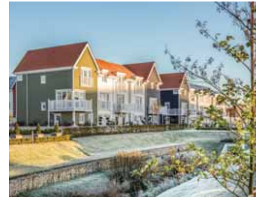
Houses Phase 1- precedent image - coloured timber weatherboard
