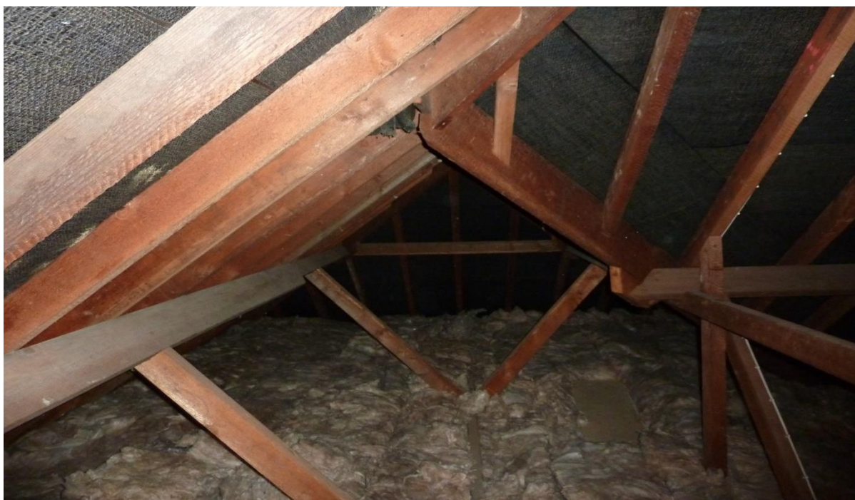
Picture 5: Showing the internal structure of the roof showing intact felt and floor insulation
