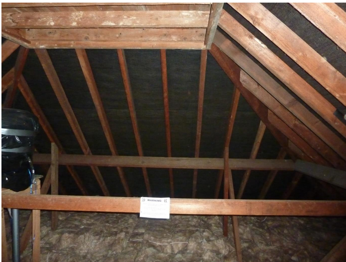
Picture 6: Showing the internal structure of the roof showing the intact felt and floor insulation.
