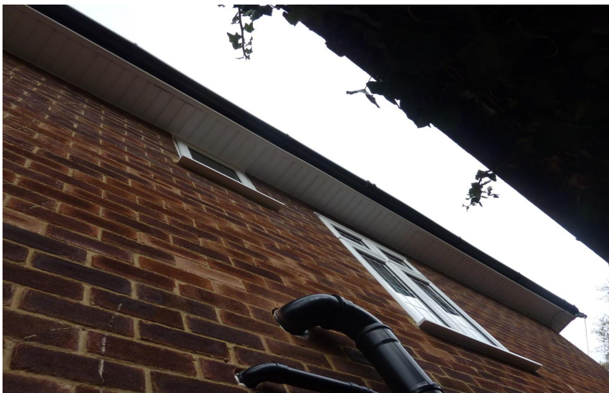
Picture 4: Showing the tight eaves made from uPVC
