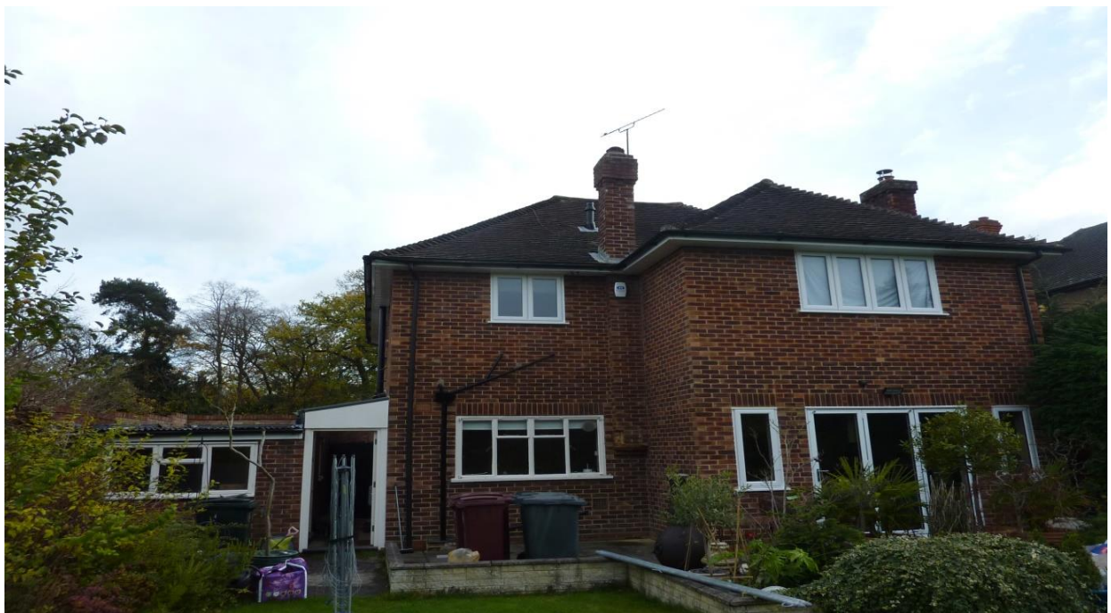
Picture 2: The rear of the property (western elevation) also showing the attached garage
