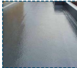
Grey liquid applied flat roof system for the main areas of flat roof across the site.
