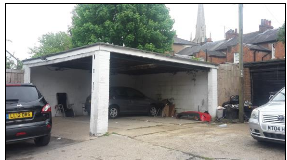
PHOTO 3 View to SE corner
