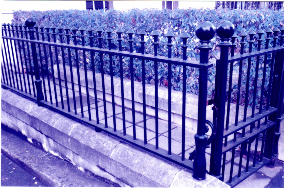
Railings at Eldon Lodge, Eldon Road / Kings Road.
