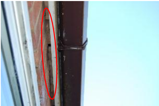
Photograph 3. A clean gap beneath the barge board fitted to the single-storey extension.
