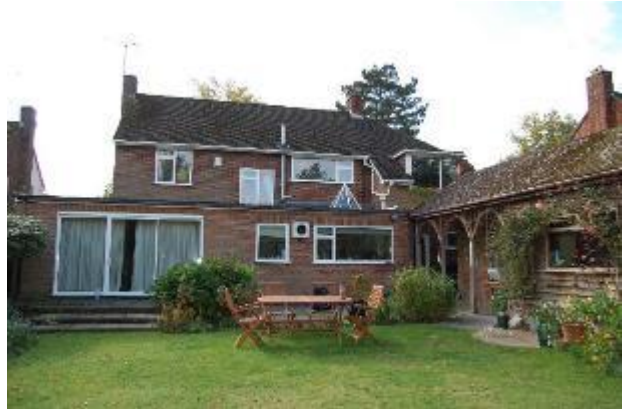
Photograph 2. The rear (northern side) of the property.
