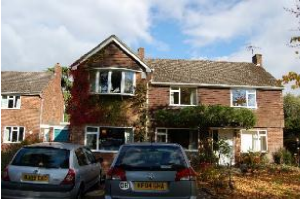
Photograph 1. 50 Chazey Road, viewed from the south.
