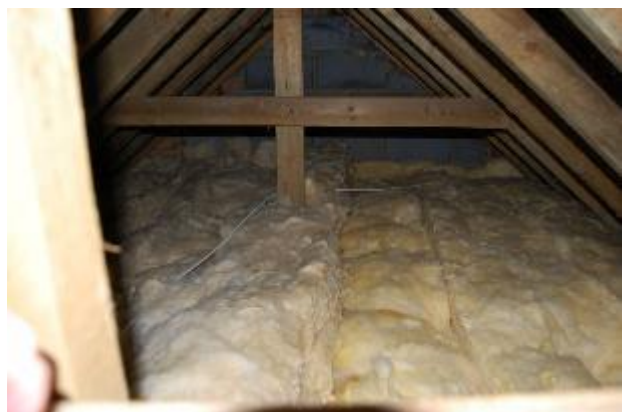
Photograph 6. The smaller loft space within the south-western corner of the roof space.
