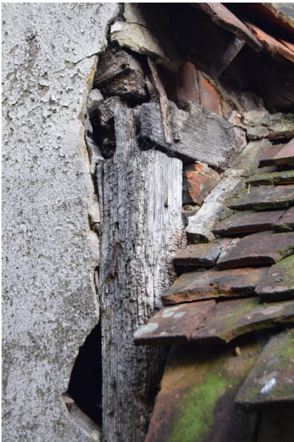
Plate 12: Corner post and wall plate of (phase 1) rear wall frame
