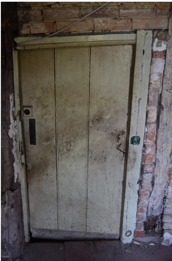
Plate 28: Planked and ledged rear door
