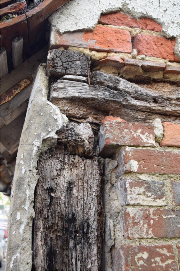
Plates 4 and 5: Detail of oak frame revealed on south gable end at wall plate/post junction
