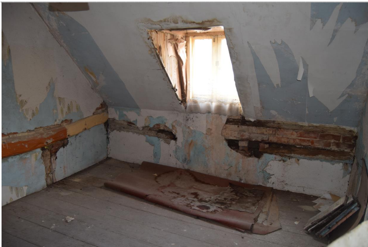
Plate 21: South bedroom, showing two wall plates on the front wall
