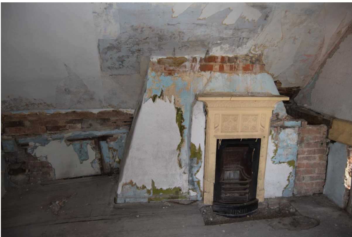
Plate 22: South bedroom, showing two wall plates and chimney on rear wall
