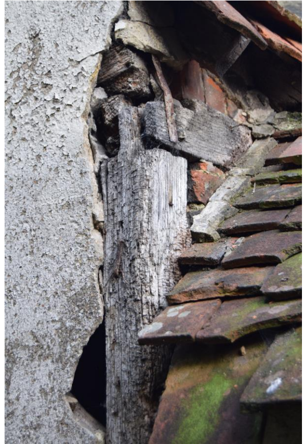
Plates 4 and 5: Detail of oak frame revealed on south gable end at wall plate/post junction
