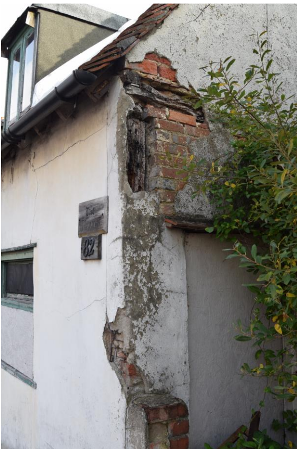
Plates 2 and 3: The south elevation exposes elements of the original oak frame
