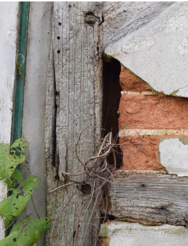
Plates 9 and 10: Detail of frame decay in north gable
