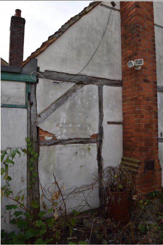
Plates 7 and 8: North elevation timber framing
