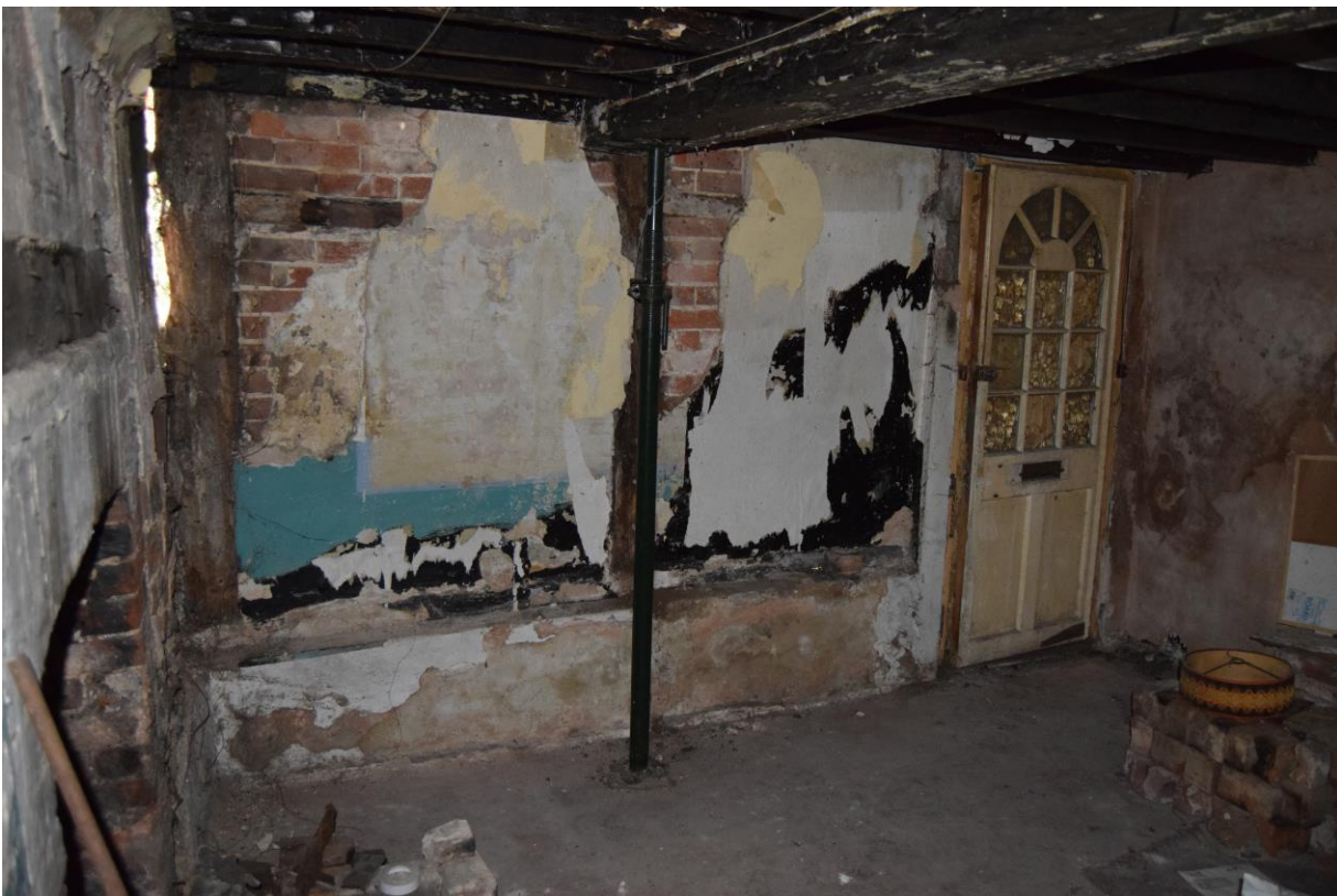
Plate 14: South room end wall showing remnants of phase 1 timber framing
