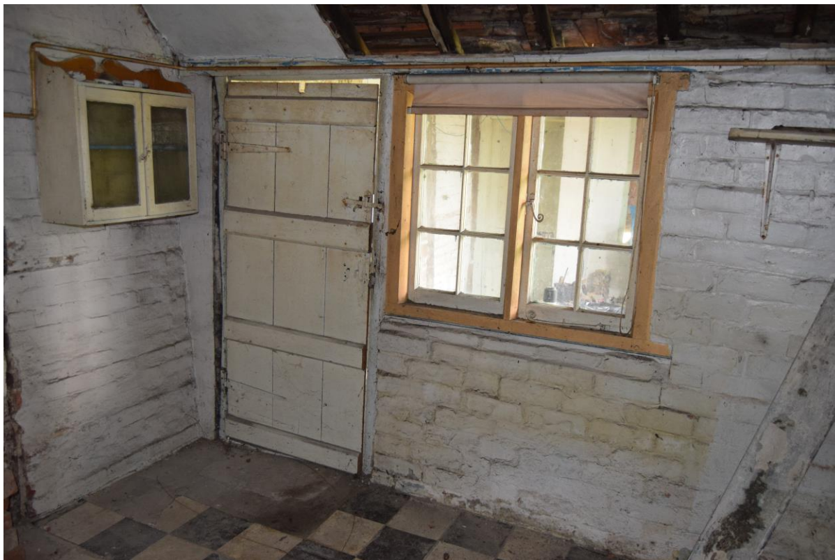
Plate 25: Interior of 19 th century extension
