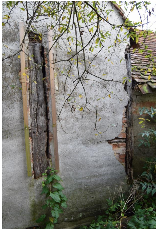
Plates 2 and 3: The south elevation exposes elements of the original oak frame
