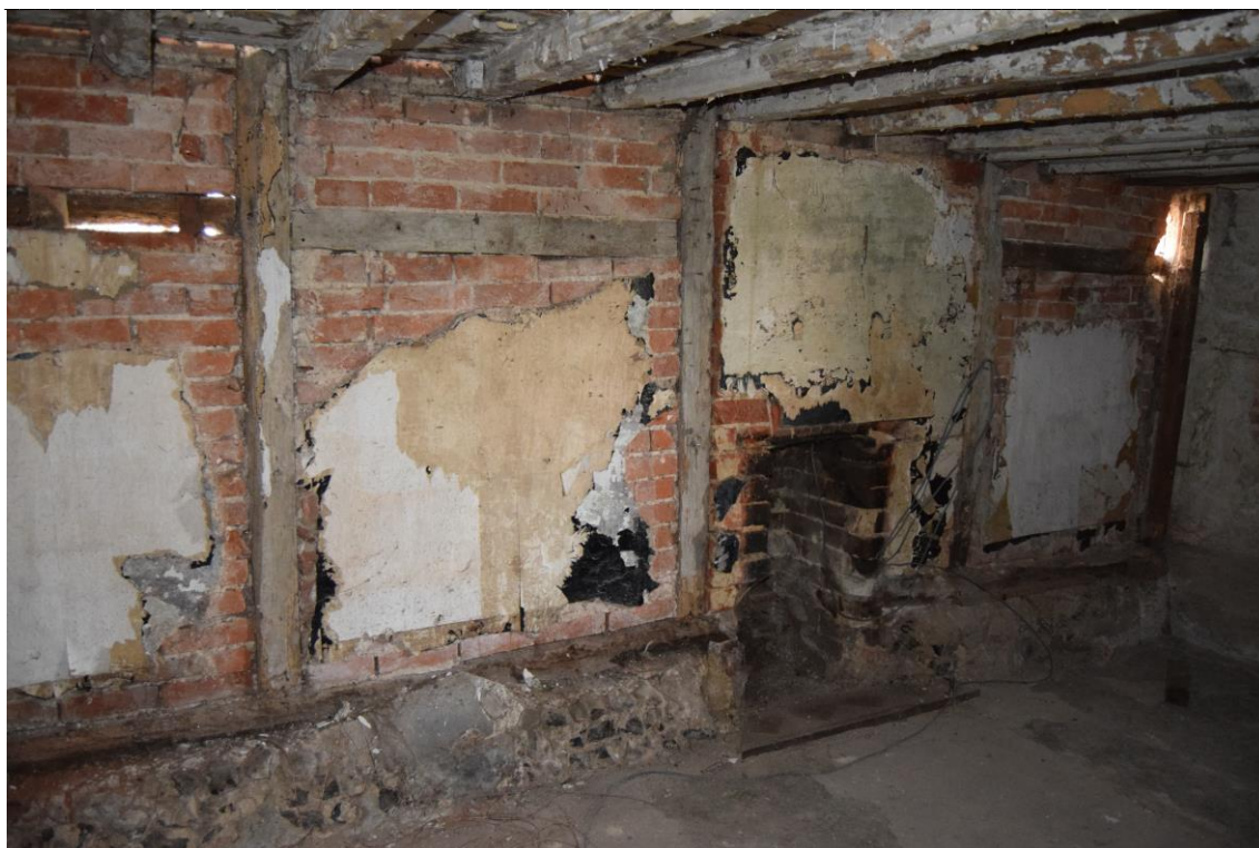
Plate 17: North room looking towards north gable end
