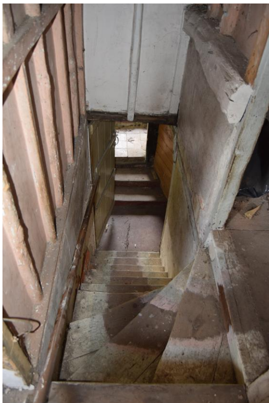
Plate 19: Staircase viewed from the top
