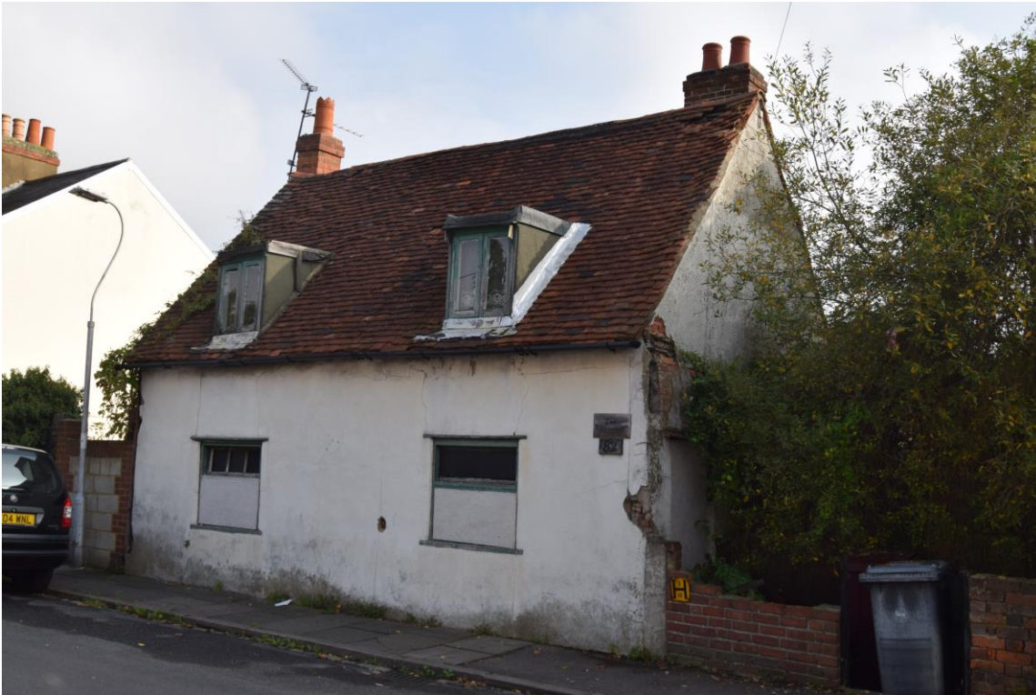
Plate 1: West and south elevations
