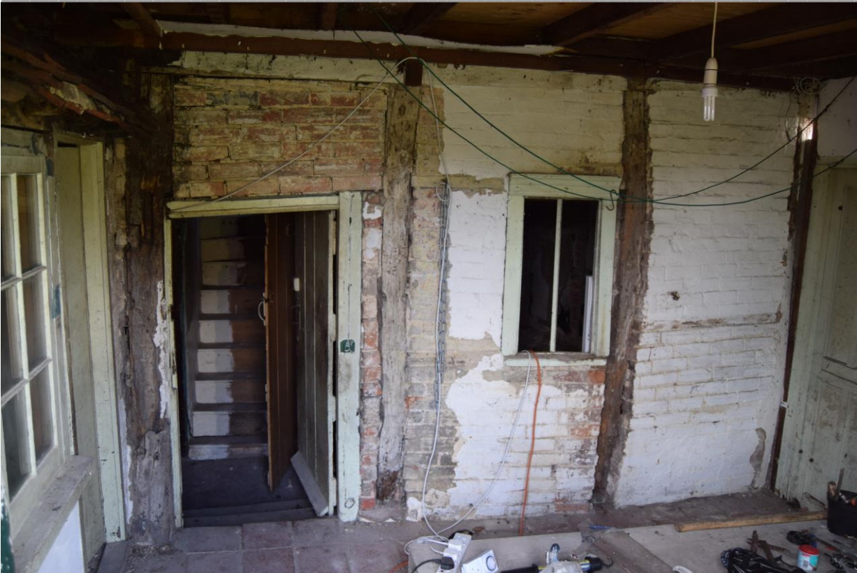
Plate 27: Interior of 20 th century flat roofed extension
