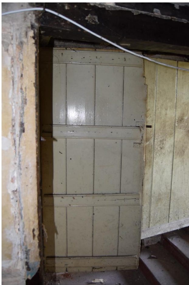
Plate 18: Ledged door at base of staircase
