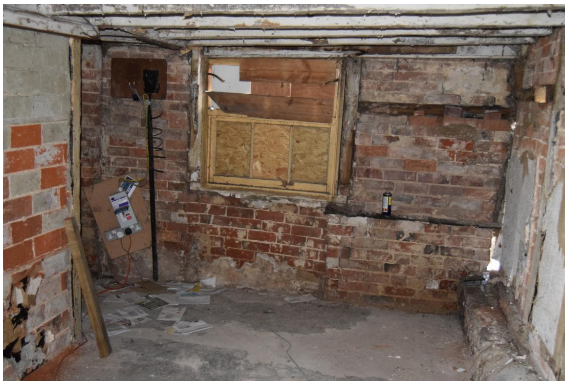
Plate 16: North room looking towards front elevation
