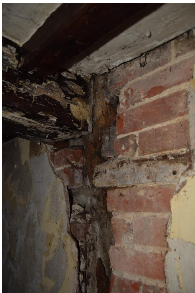
Plate 15: Junction of south room spine beam against south gable end
