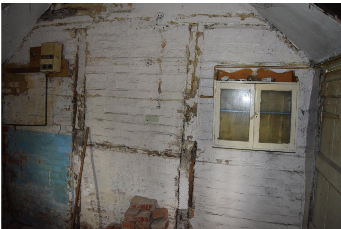
Plate 26: Rear wall of original building from inside 19 th century extension
