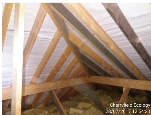
Figure 6: Newer roof section with BRM
