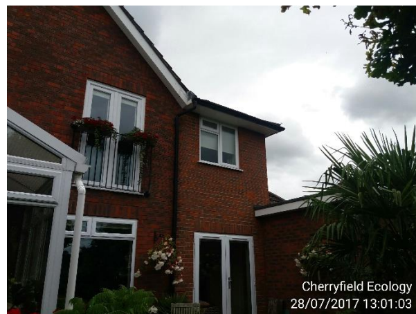
Figure 4: Flat roofed extension
