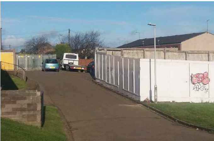
Access off Thurso Close, western boundary of the site.
