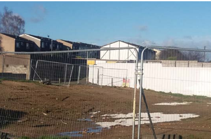
Site viewed from the south.
