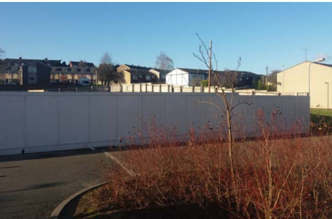
Site eastern boundary adjoining main footpath.
