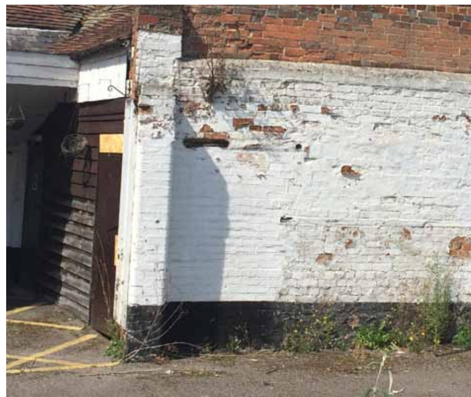
Fig.11: Evidence of lintel can be seen in the rear elevation
