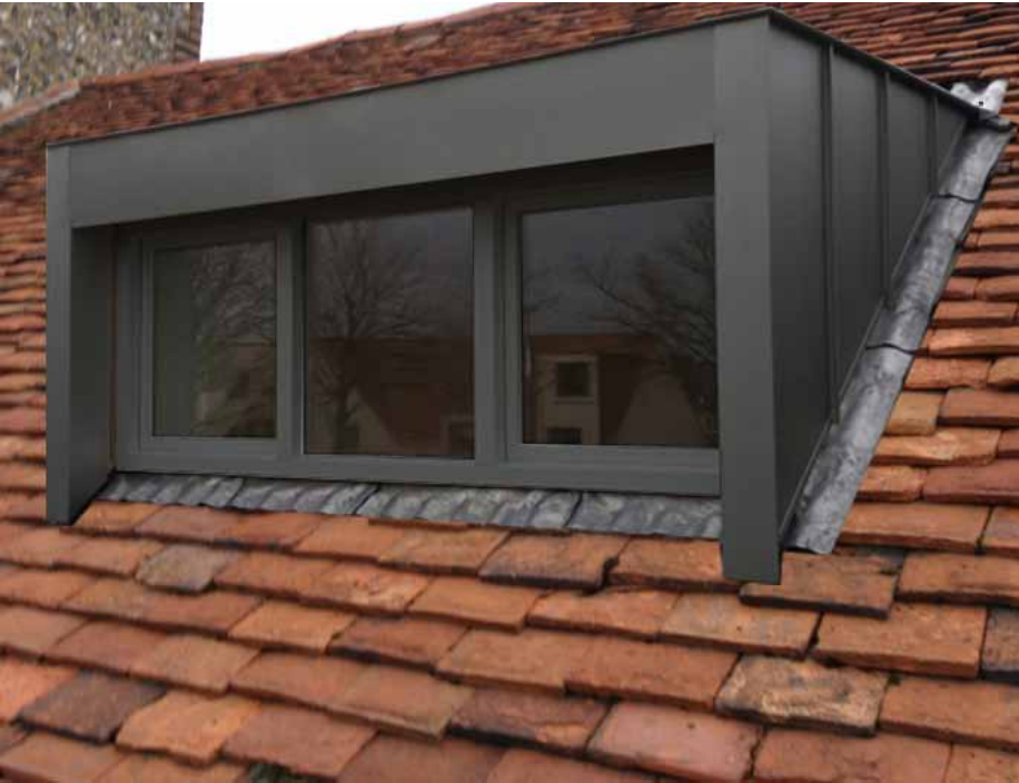
Fig.42: Metal clad dormer with grey window frame and reclaimed red clay roof tiles
