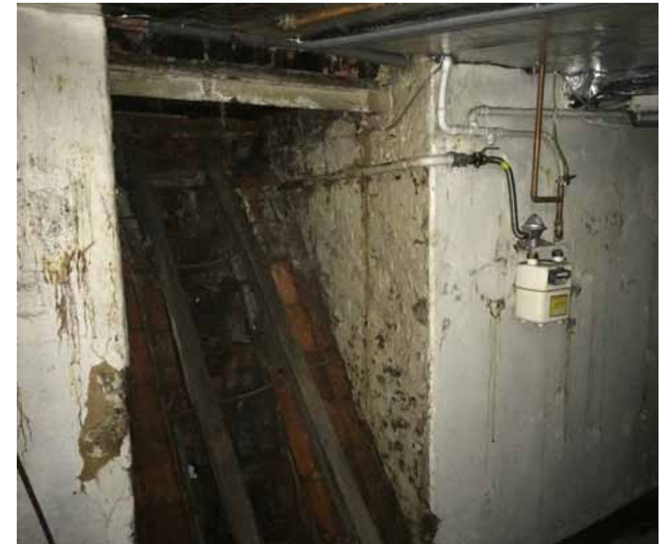
Fig.13: Existing basement with low head height and access ramp to Crown Street
