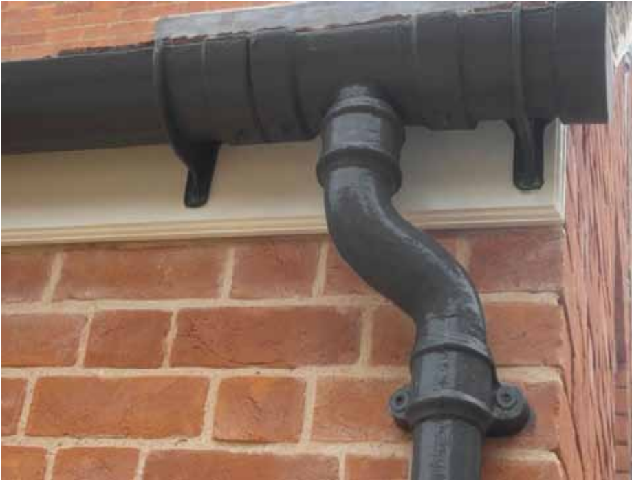
Fig.41: Black painted cast iron rainwater goods
