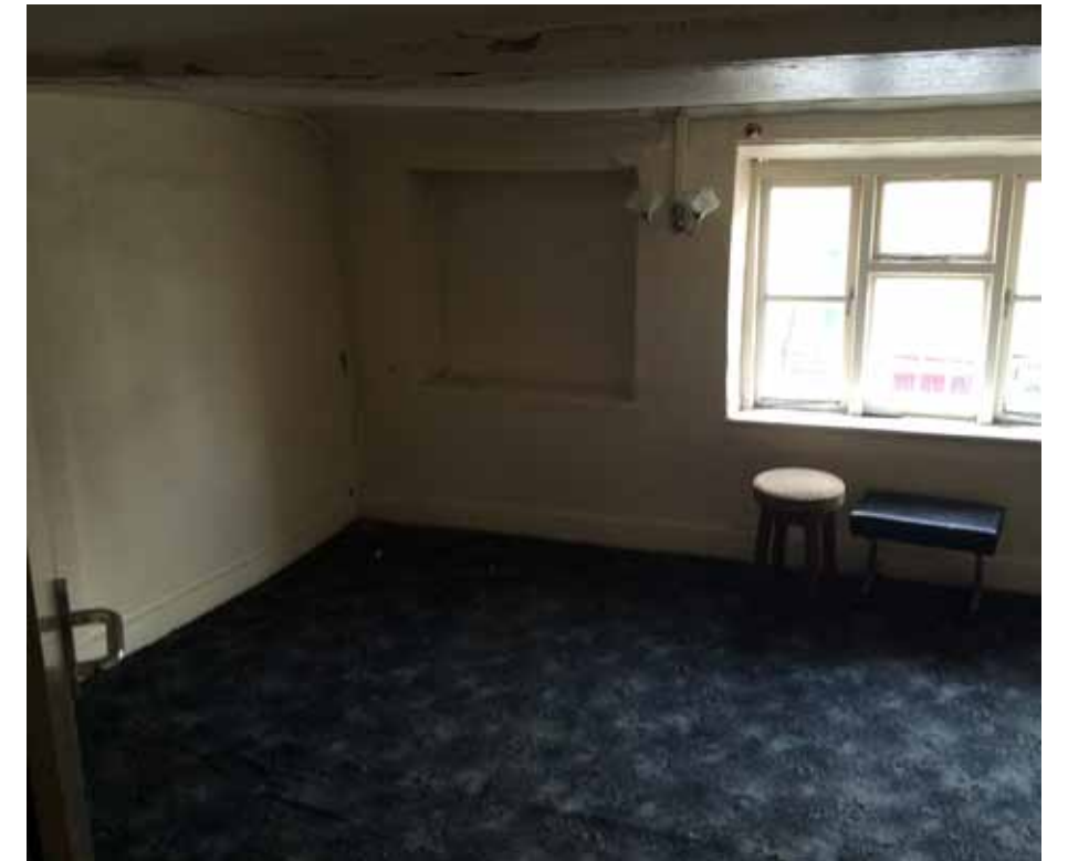
Fig.17: Existing first floor room with low head height
