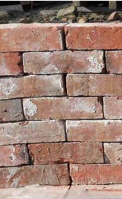
Fig.43: Reclaimed red bricks
