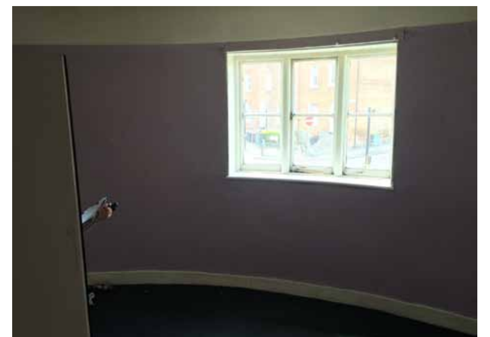
Fig.18: Existing first floor corner room overlooking Southampton Street and Cronw Street
