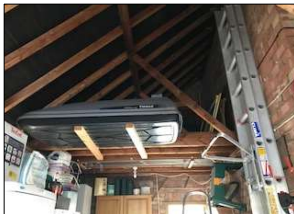
Photo 15: Integral garage beneath catslide roof. Bitumen lining visible.
