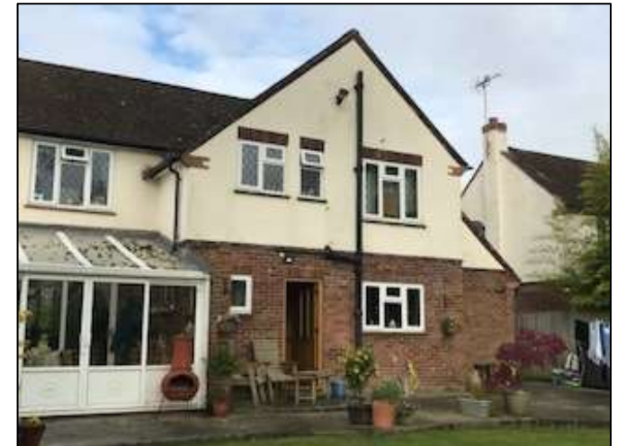
Photo 3: One of the additional pitched roofs at the rear (north-east elevation).
