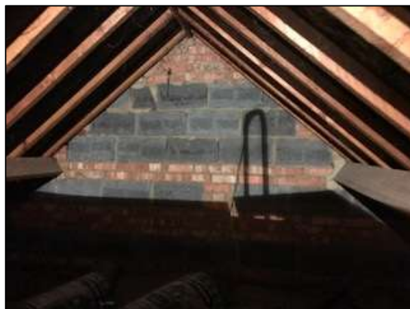
Photo 13: Interior of additional pitch within L1.
