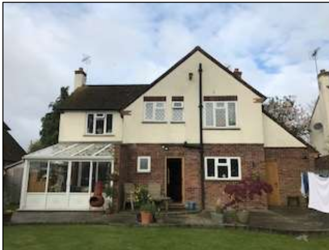
Photo 2: Rear (north-east) elevation of B1.
