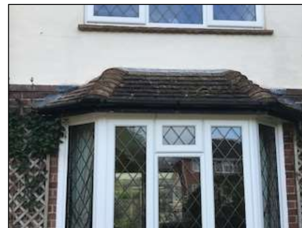
Photo 6: Clay tiles above south-west corner bay window.
