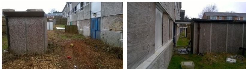
Plate 4.9: View of the Outbuildings.
