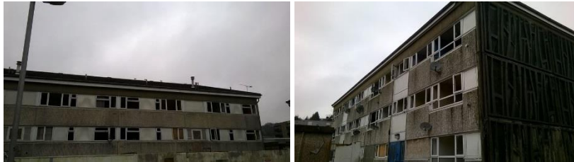
Plate 4.5: View of Buildings 2 and 3 Respectively.
