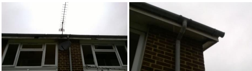
Plate 4.2: Gaps were Present where the Soffits of Building 1 were Broken.
