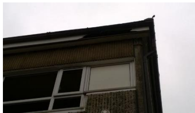
Plate 4.6: Broken Soffit of Building 3 (Block 12).
