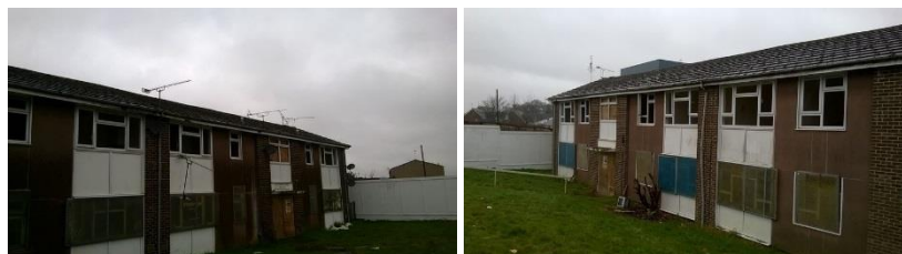
Plate 4.1: View of Building 1 (Blocks 24 and 26).
