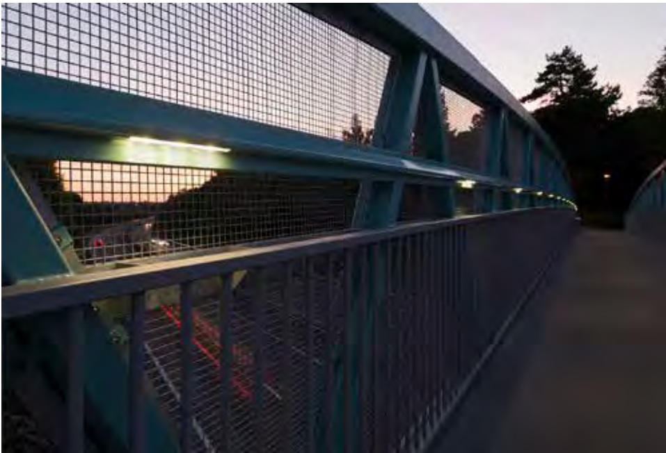
Figure 118. Bridge deck lighting concept (DW Windsor Garda LED Rail Lighting, copyright DW Windsor)
