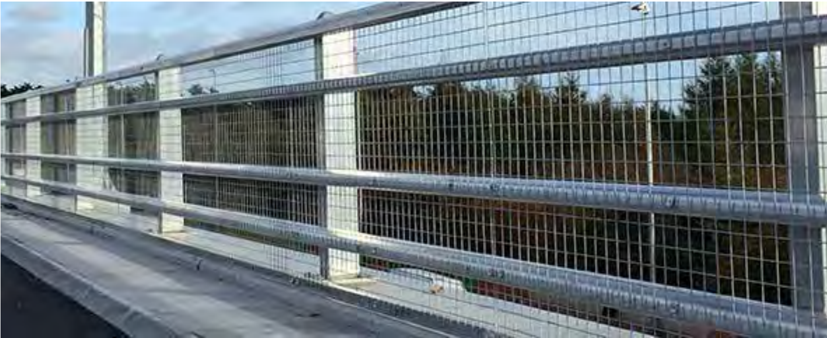
Figure 94. Balustrade rail with mesh infill
