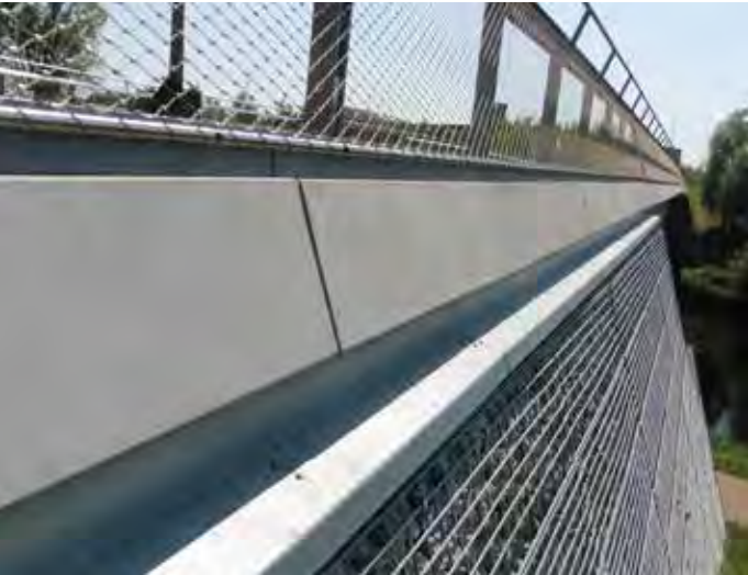
Figure 98. Example of gabion clad abutment at junction with concrete deck
