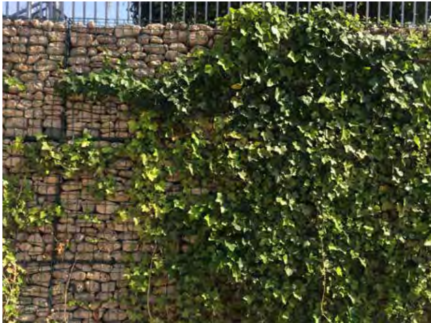
Figure 95. Example of gabion wall
