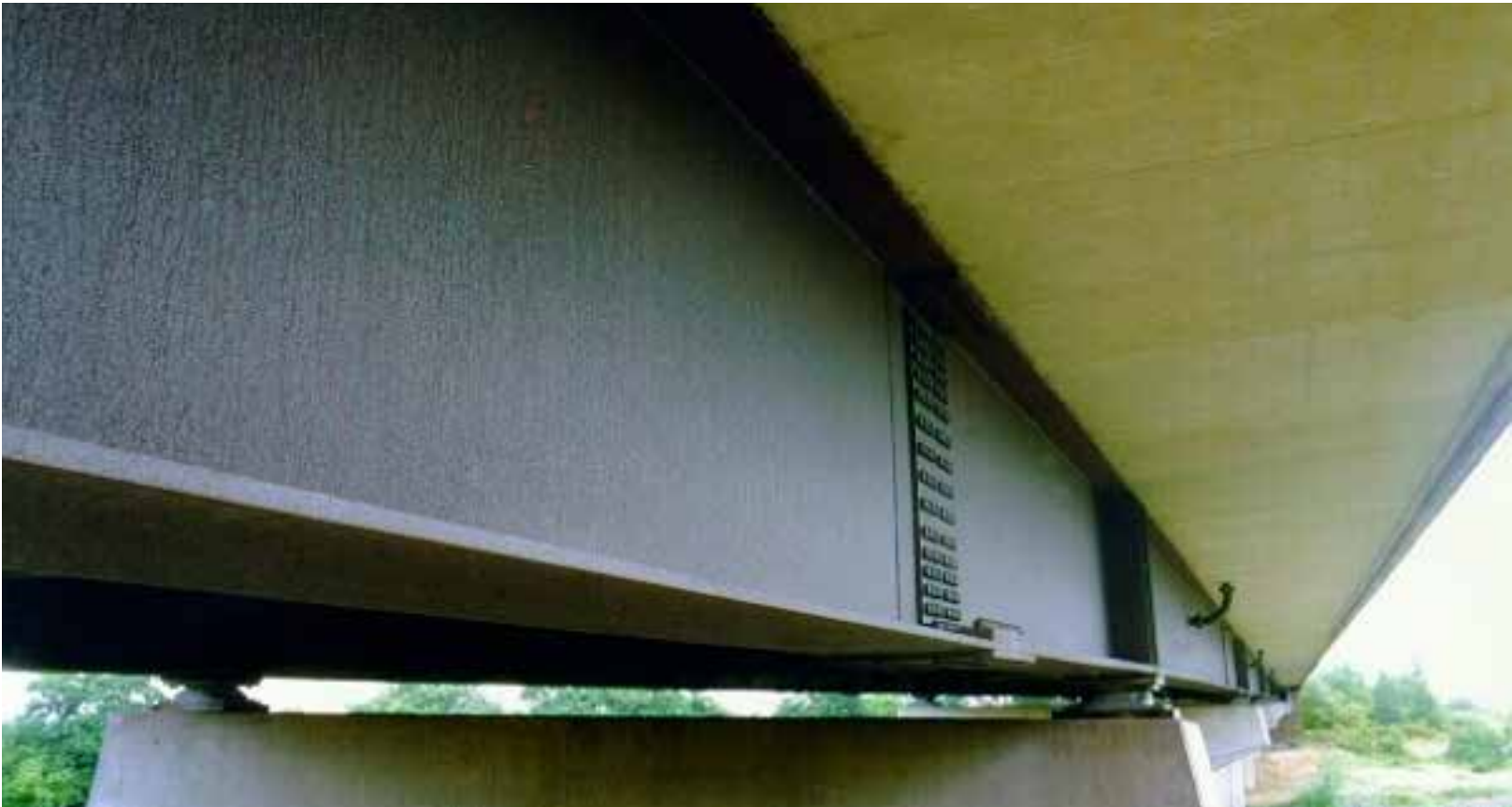
Figure 93. Example of weathering steel finish
