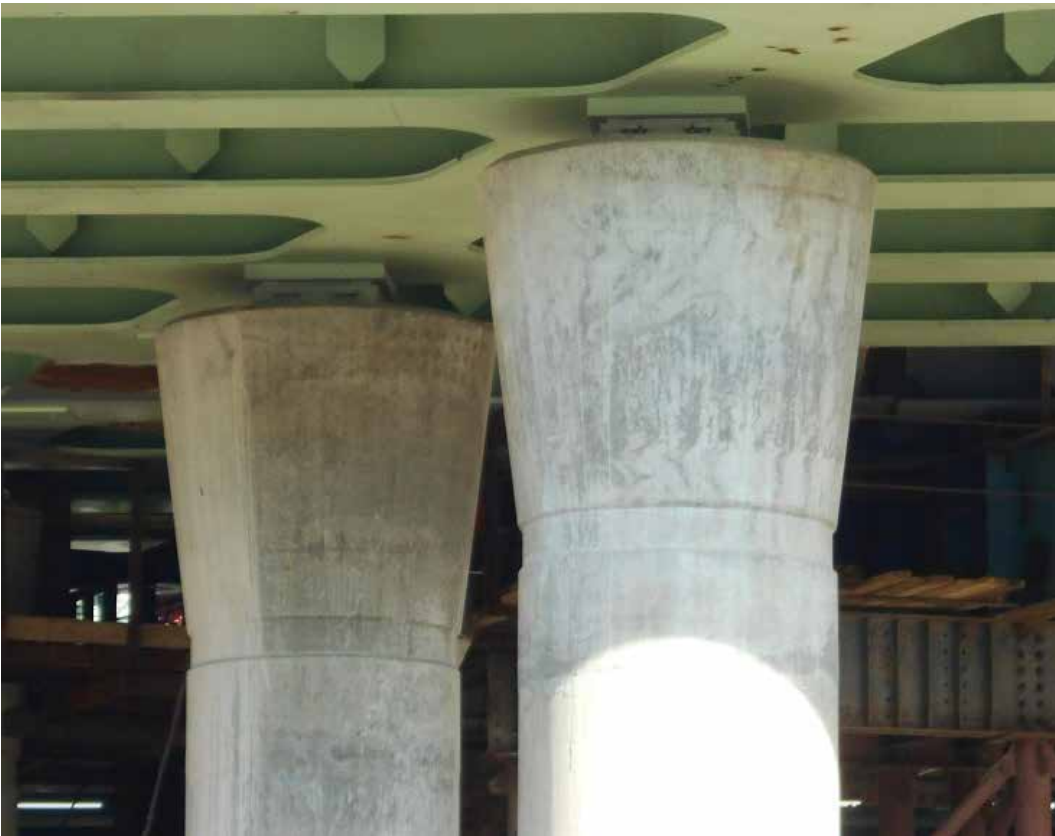
Figure 63. Example of tapered column head
