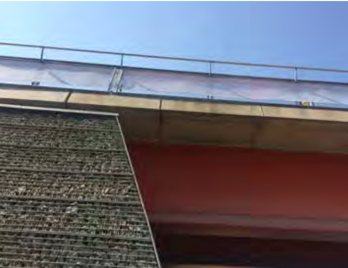
Figure 100. Example of gabion clad abutment at junction with concrete deck
