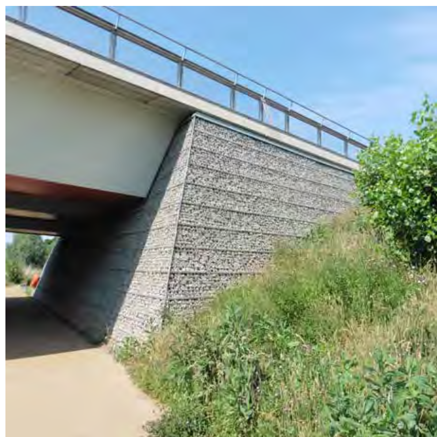
Figure 61. Example of a bridge abutment with gabion wall
