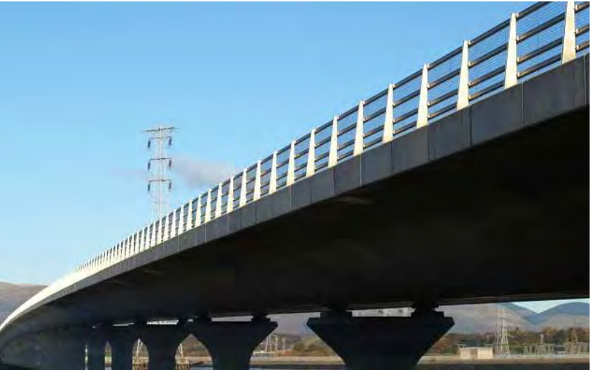
Figure 101. Example of railing with horizontal rails emphasizing curving form of viaduct
