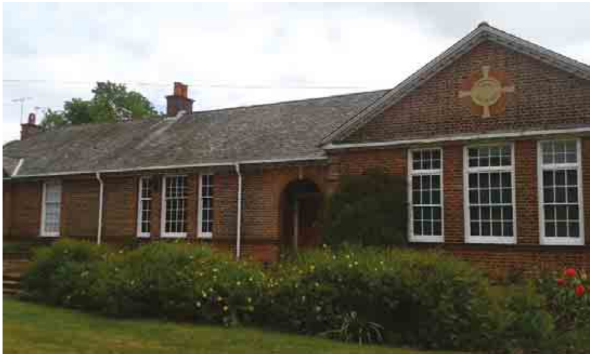
Photograph 16b: Single storey building next to Pearson's Court
