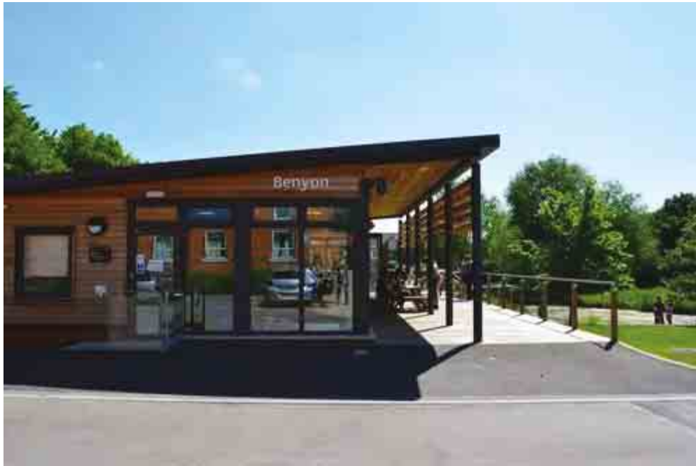
Photograph 24: Benyon Hall JCR
