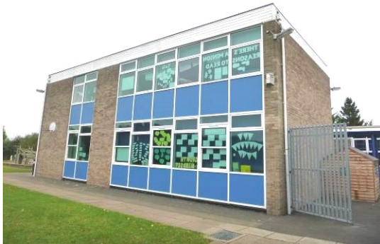
21. One of the two storey buildings to the northern end of the school.
