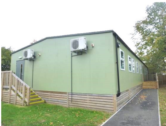
25. Building 6 situated to the north of the school with a flat roof
