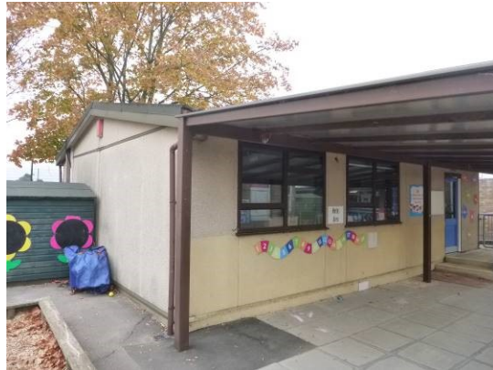
16. Nursery building situated to the south west of the school with prefabricated walls and a pitched roof.
