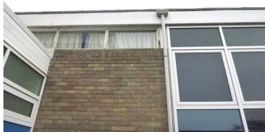
24. ICT building with the metal overhanging on the roof.
