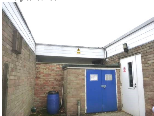
18. Southern section of the school with single storey flat roof buildings.
