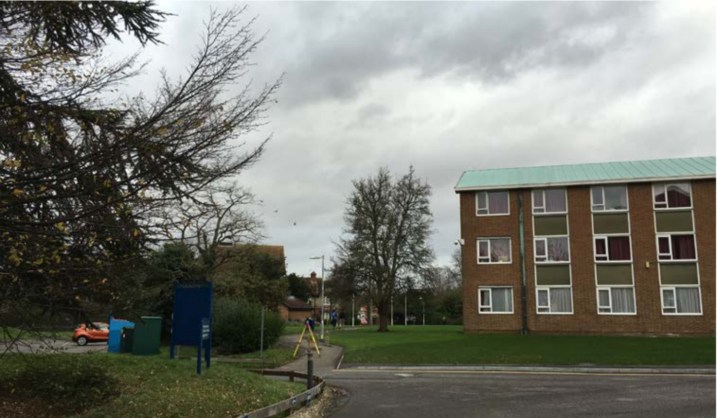
New Court looking north east towards Creighton Court
