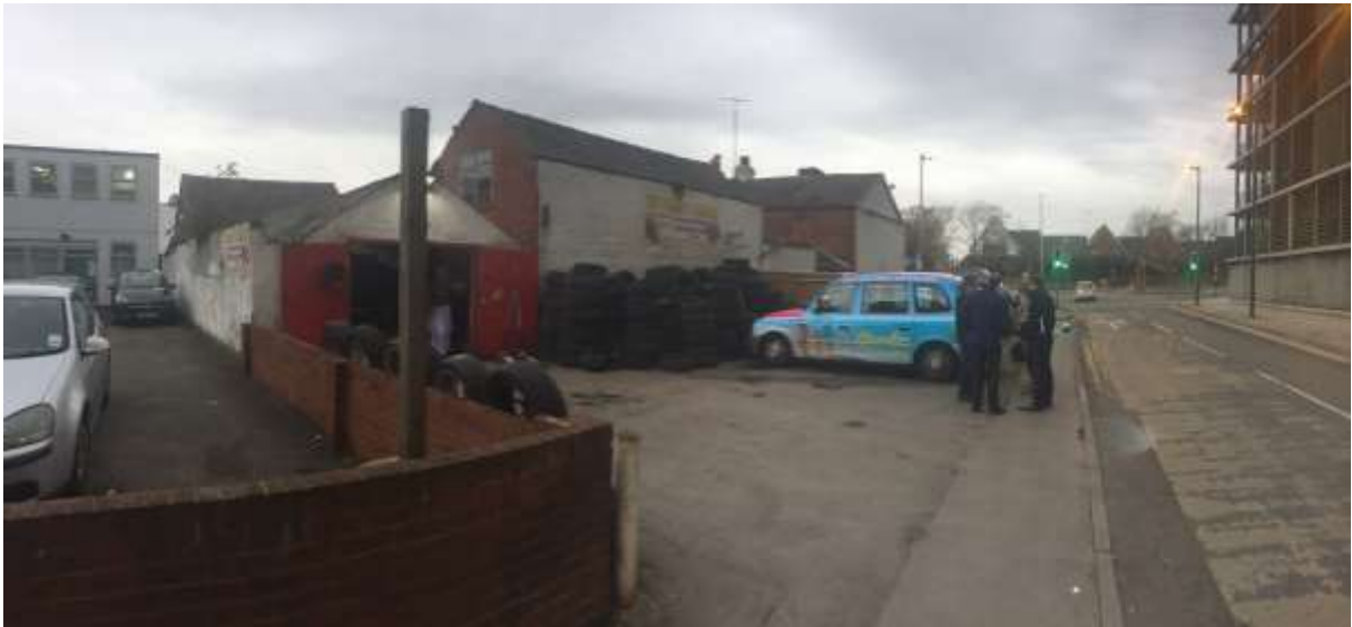
Fig 3: East Elevation and main entrance to previous tyre company
