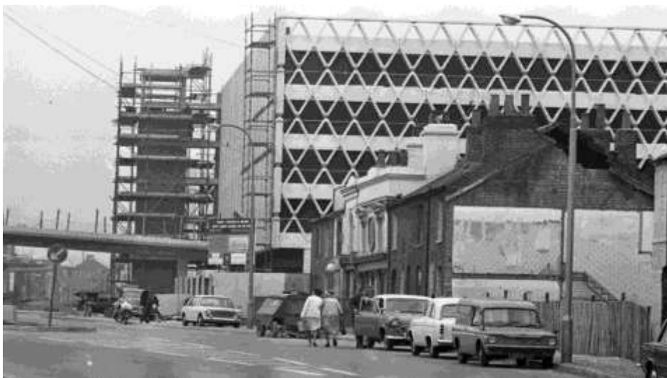
Fig 8: Construction of Chatham Street Car Park, 1968
