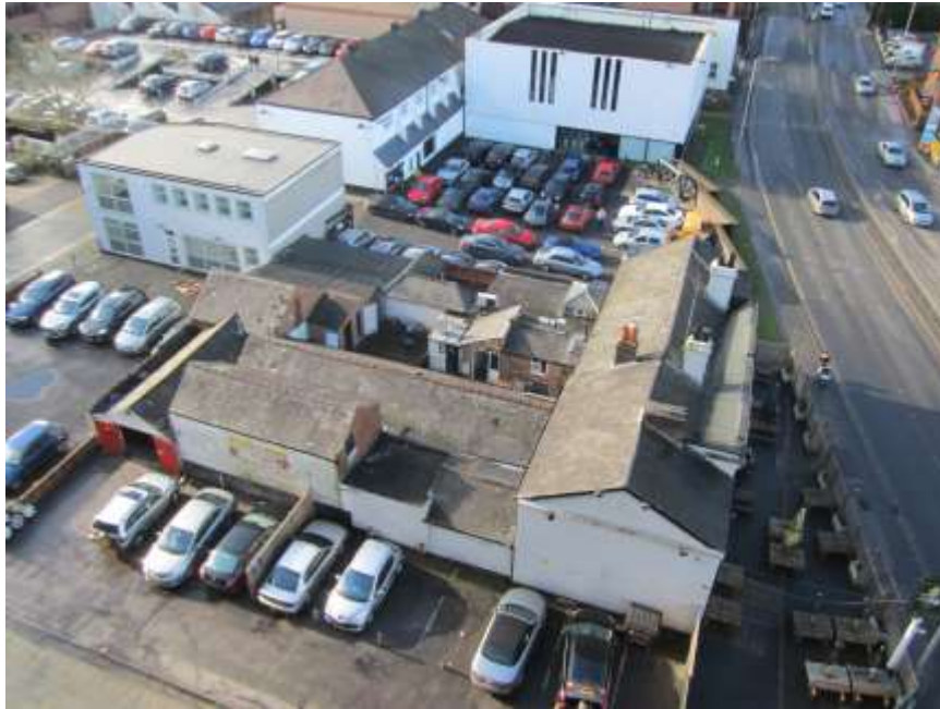
Fig 5: View from the adjacent QPark multi-storey car park
