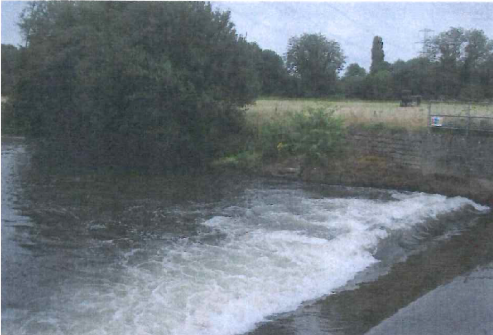
e. Theale Crump Gauging Weir
