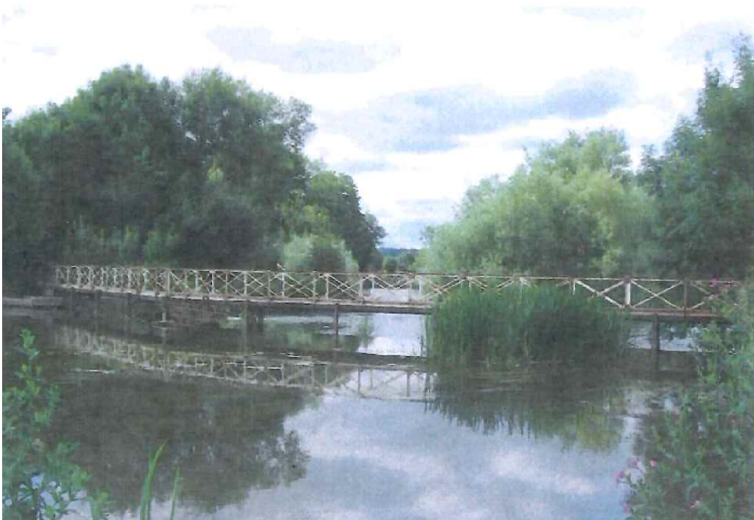
d. Sulhamstead Weir Head of Holy Brook
