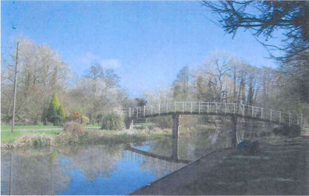
g. Milkmaids bridge at Lock 104
