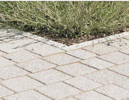
Concrete paving to public realm
