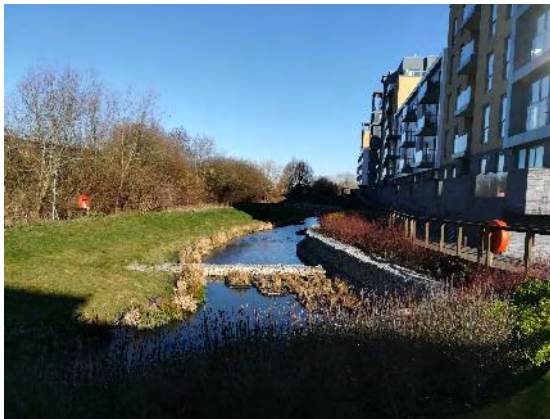
Photo 5. Recently constructed pond along Foudry Brook corridor, adjacent to the north.
