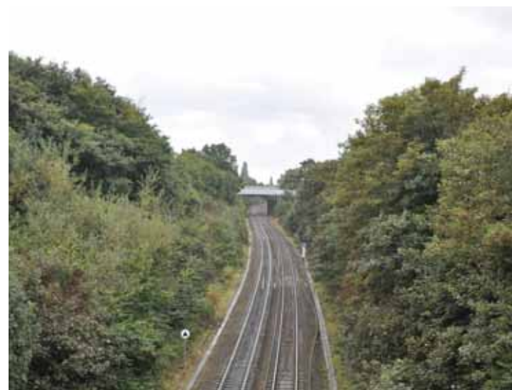
Figure 8: View from bridge towards country end showing Bath Road Overbridge
