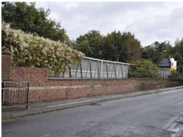
Figure 9: Low mileage parapet with modern adjacent footbridge
