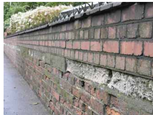
Figure 14: Close up of low mileage parapet
