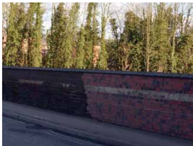
Figure 13: Detail of high mileage parapet with anti-climb spikes
