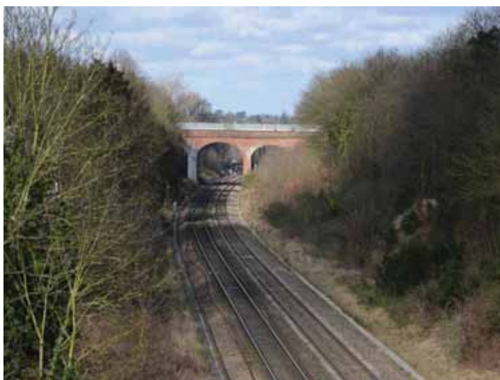
Figure 7: High mileage face seen from Bath Road Overbridge
