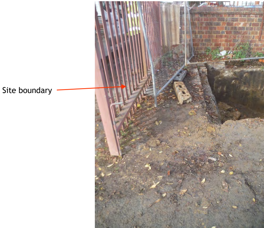
Plate 2: Photograph showing proximity of concrete chamber to site boundary and public footpath.
