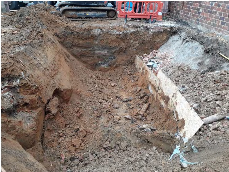
Plate 4: Photograph of completed excavation looking south west.
