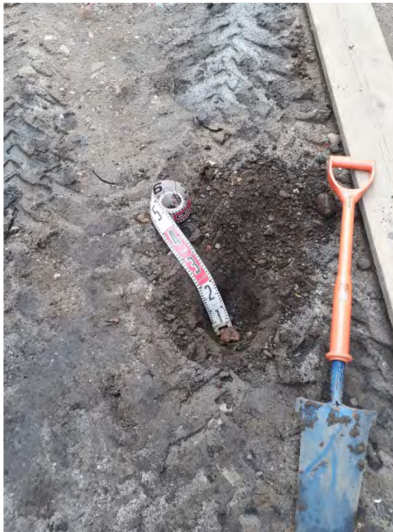
Plate 9: Hand dug pit HD03 undertaken in Plot 2 / 3, confirming 300mm of capping.
