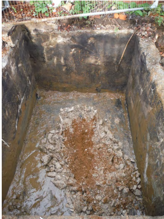
Plate 1: Waste oil tank concrete chamber following removal of tank. Concrete base broken out and underlying soils exposed.
