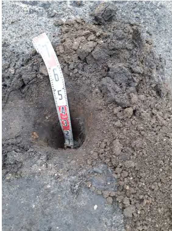
Plate 7: Hand dug pit HD01 confirming placement of 600mm of capping in Plot 4.
