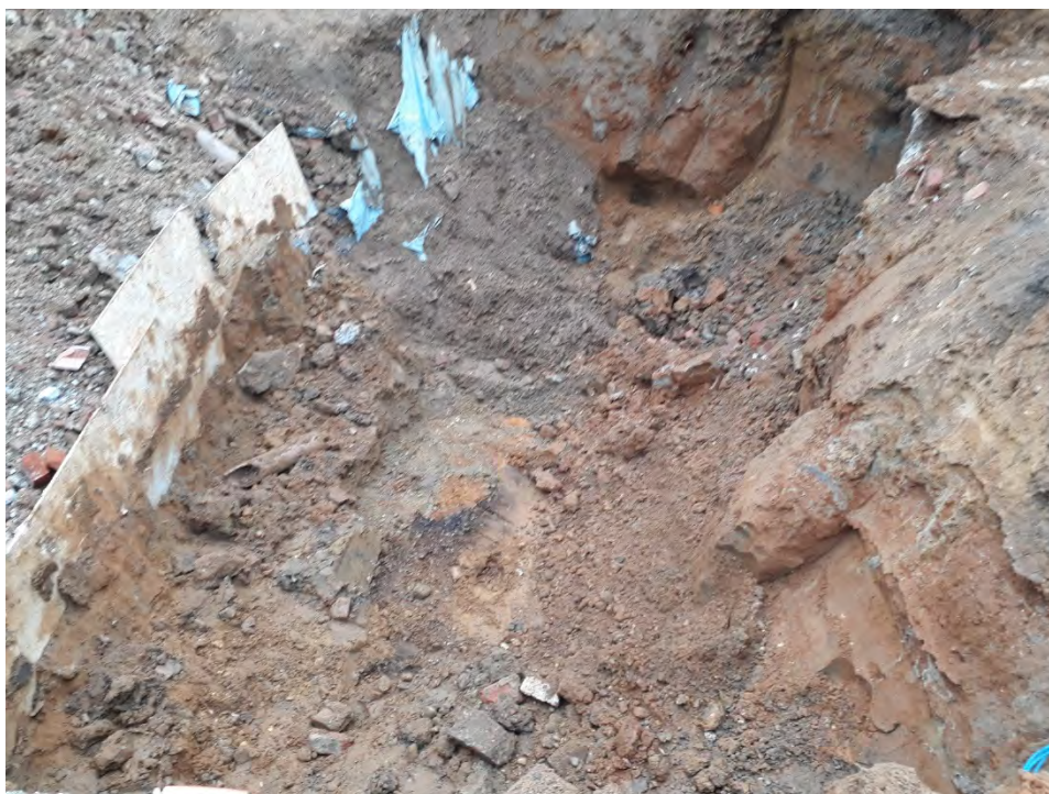
Plate 6: Photograph of excavation looking north east
