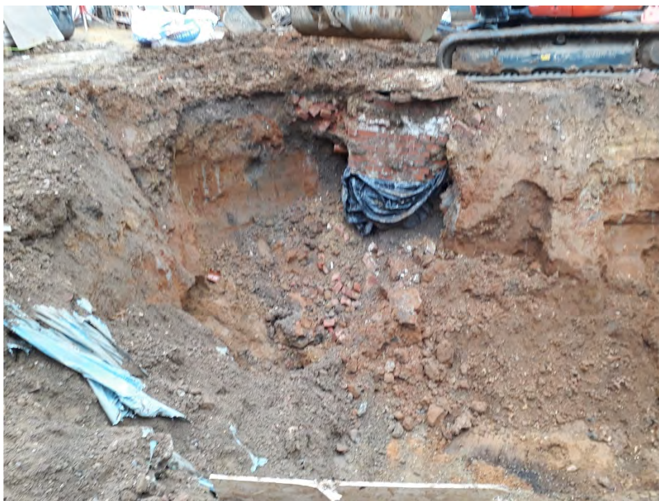
Plate 5: Photograph of excavation - Face (F3)
