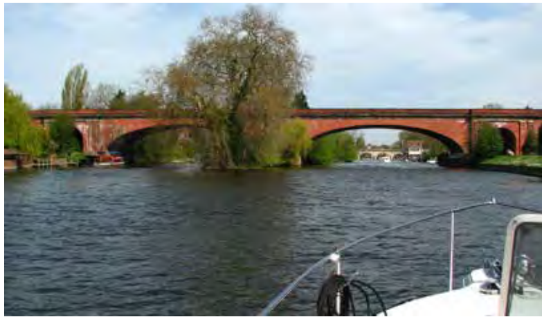
Figure 30. Maidenhead Railway Bridge
