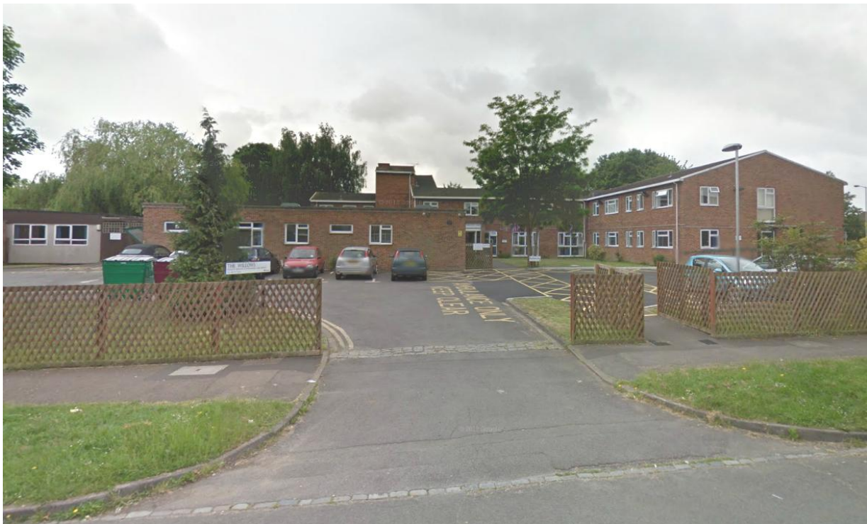
View of The Willows Care Centre from Hexham Road
