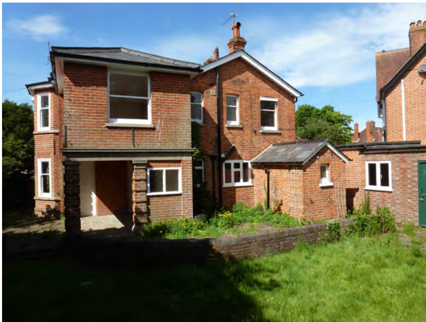
Fig. 2: Rear view of existing 25 Redlands Road
