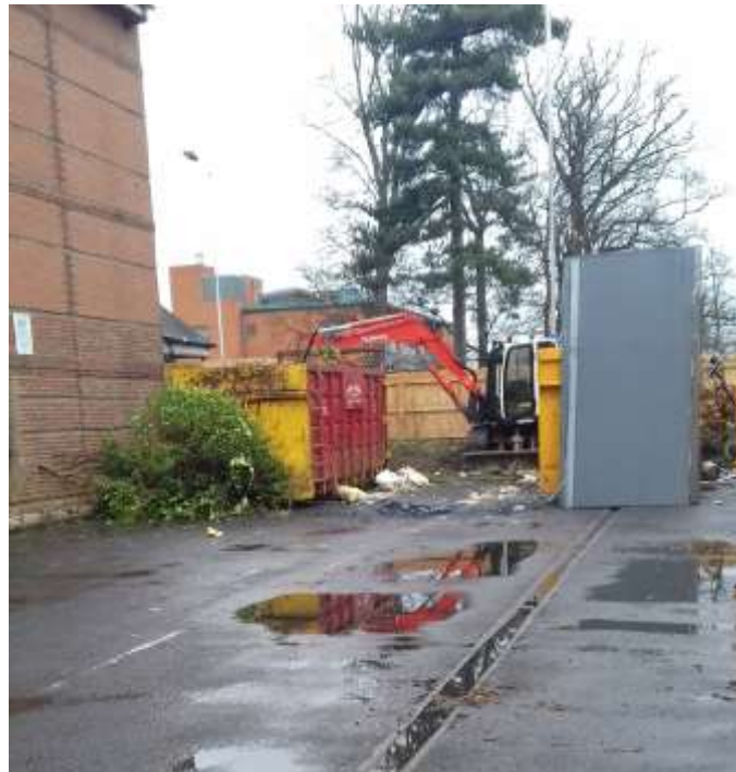
PLATE 1 – LOOKING ACROSS THE SITE TOWARDS WASTE STORAGE AREA
