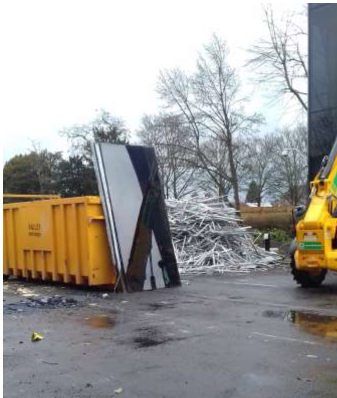
PLATE 4: WASTE STORAGE FOR THE ADJACENT SITE
