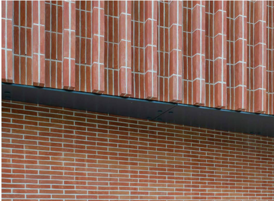
Example of 50mm high brick : East Ham Customer Services Centre / Library
