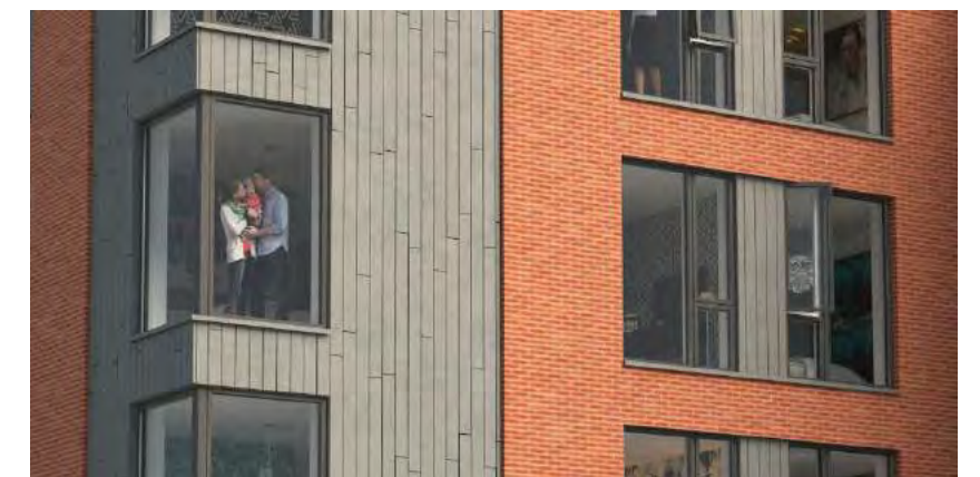
Solid window panel removed to improve natural light
