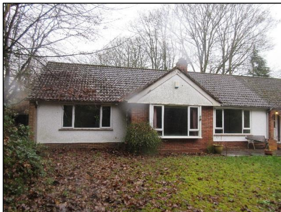
Photograph 17: Western half of southern elevation
