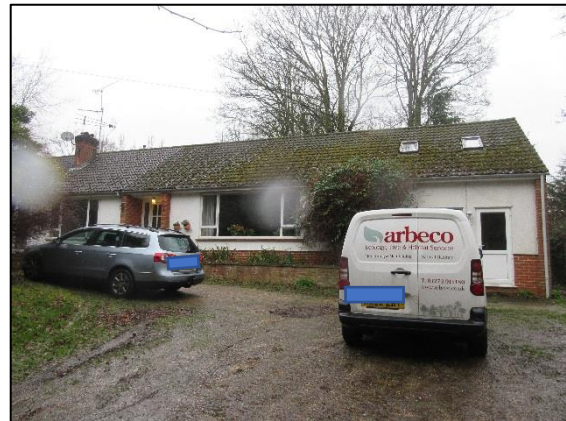
Photograph 16: Eastern half of southern elevation
