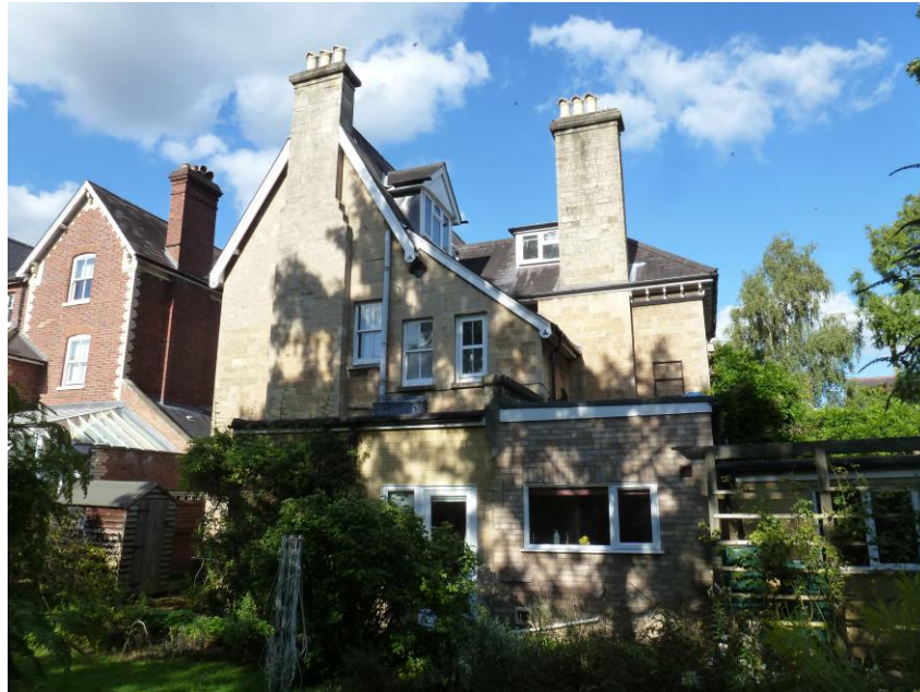
Fig.3: View of rear of 26 Alexandra Road from back garden.
