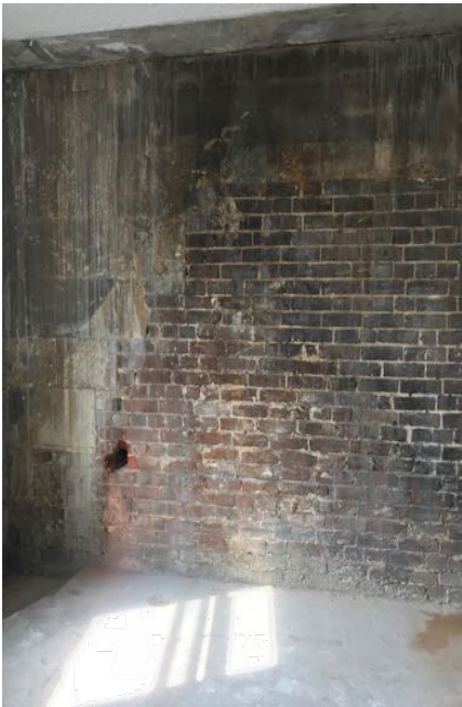
EXISTING BRICKWORK AND STONE FROM ORIGINAL DEVELOPMENT CLEANED AND MADE A FEATURE WALL
