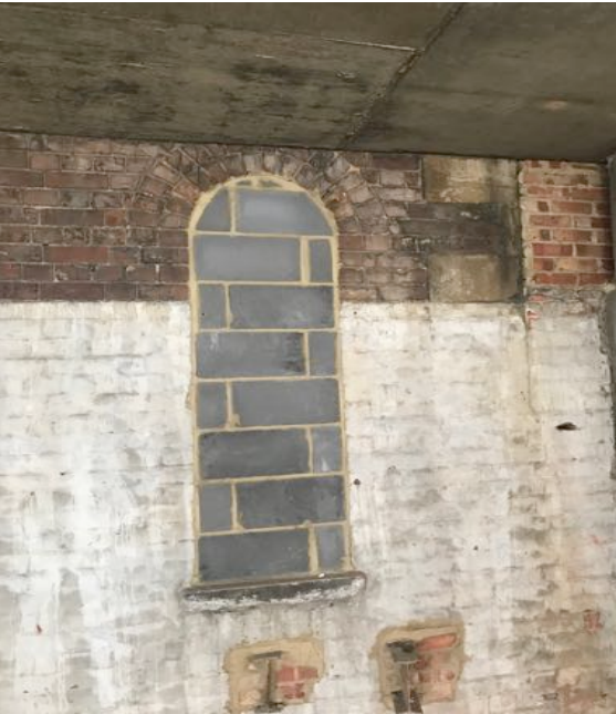
EXISTING FEATURES RETAINED AND REFURBISHED
