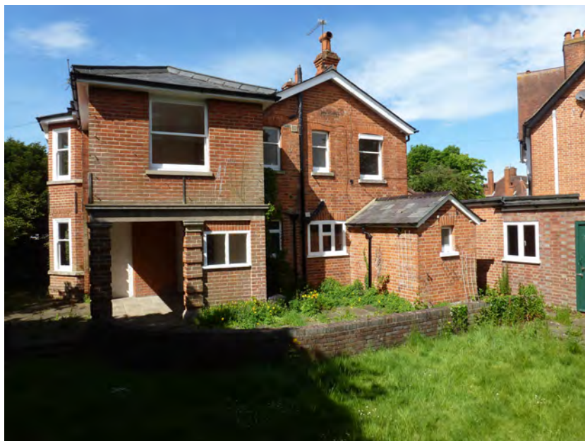
Fig. 2: Rear view of existing 25 Redlands Road
