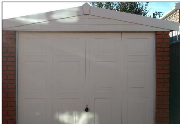
Photo 6: B2 Eastern elevation
