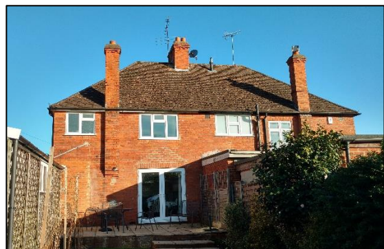
Photo 2: B1 Western elevation
