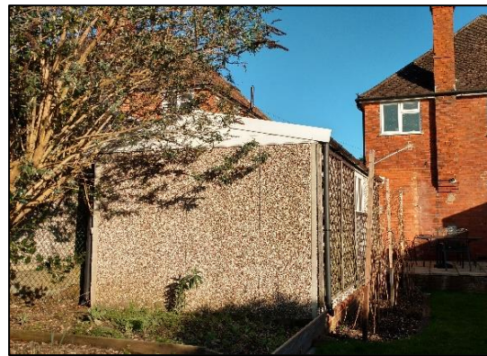
Photo 7: B2 Western elevation
