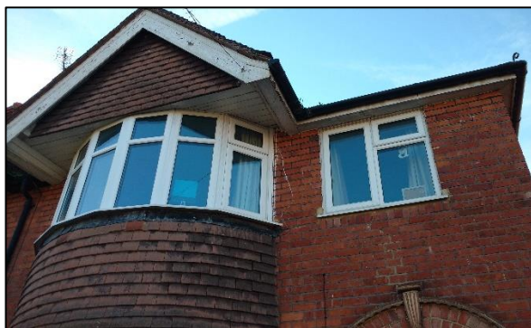
Photo 1: B1 Eastern elevation
