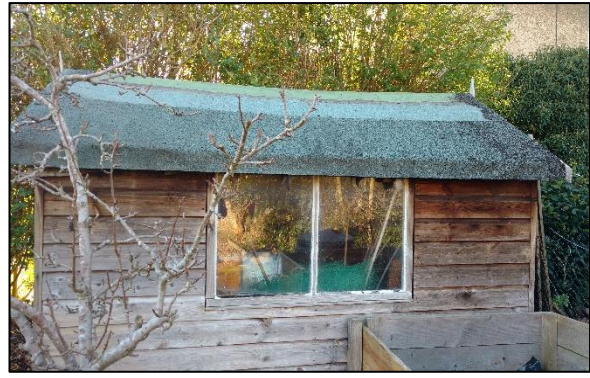
Photo 9: B3 Eastern elevation
