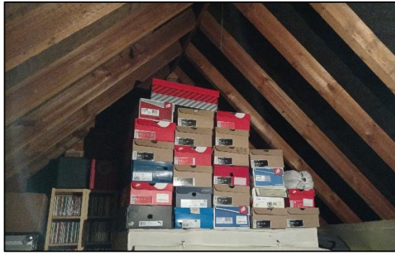
Photo 4: B1 Interior void
