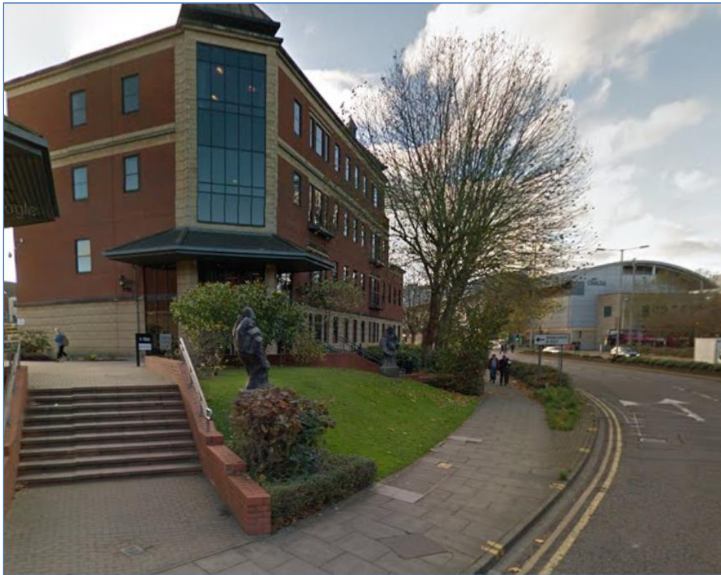
Figure 1: View of New Century Place 1 from Queen's Road
