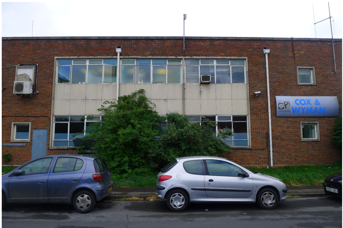
A1.13 The south end of the west elevation
