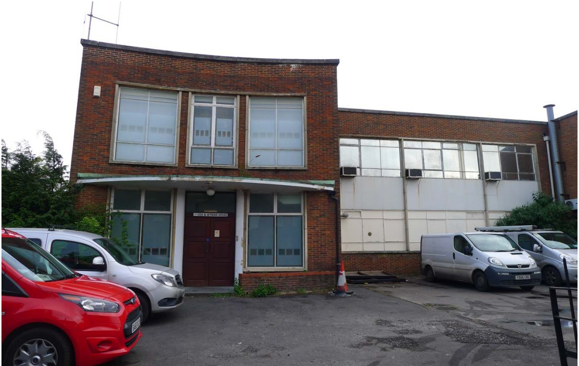
A1.2 The middle of the south elevation
