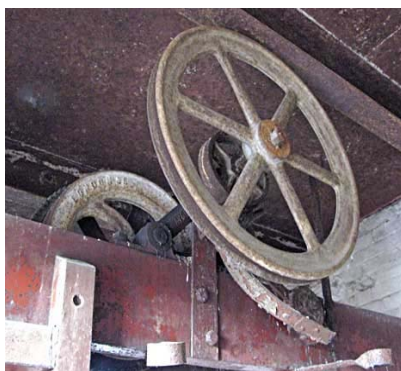
Figure 12: Victorian lift mechanism in the NE stairwell,
