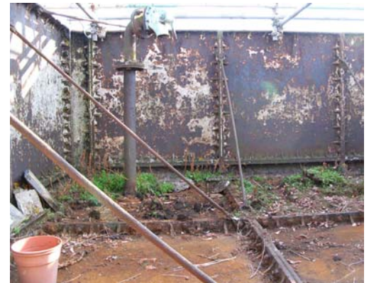
Figure 14: Interior of the cast iron tank
