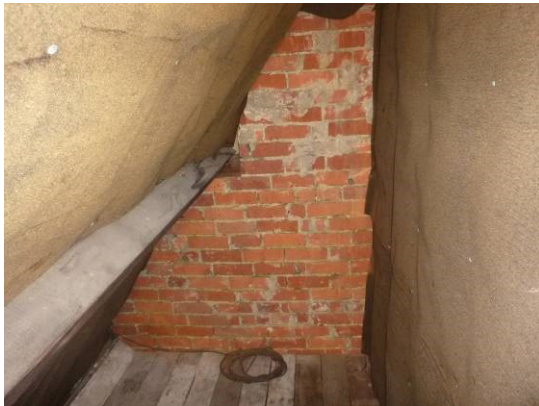
21. Brickwork at end of rear eaves space.
