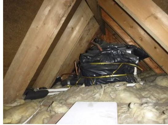
20. Boarded gable toward rear behind water tank.
