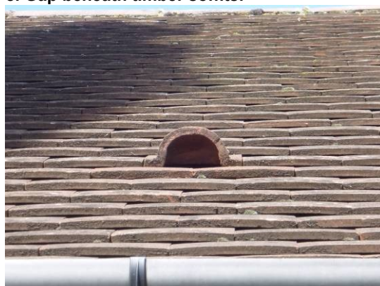
10. Vent on rear extension.
