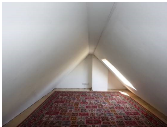
14. Internal view converted loft space.
