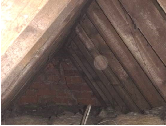
19. Brickwork intact at front facing gable.
