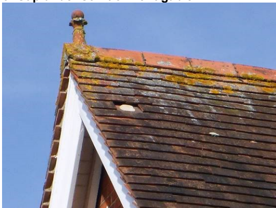
5. Missing tile at front gable
