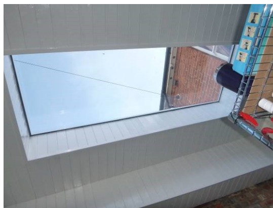
16. Skylight above pantry space.
