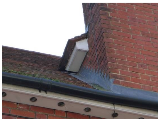
12. Lead flashing tight around chimney.
