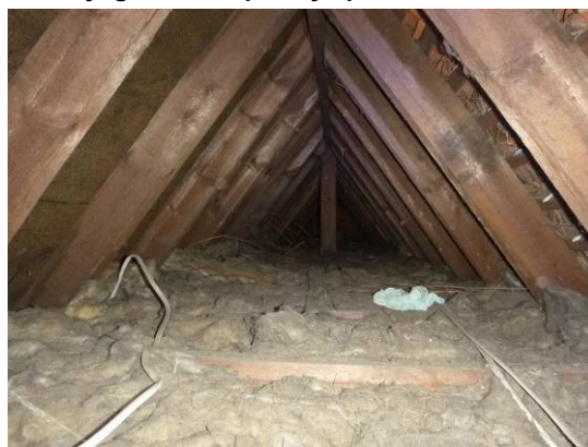
18. Main roof space half lined with bitumen felt.
