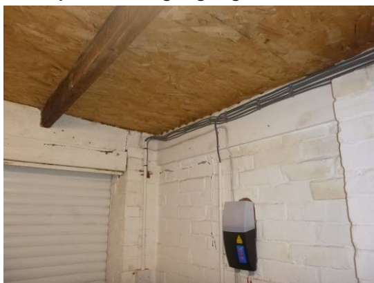
17. Polystyrene fittings at eaves.
