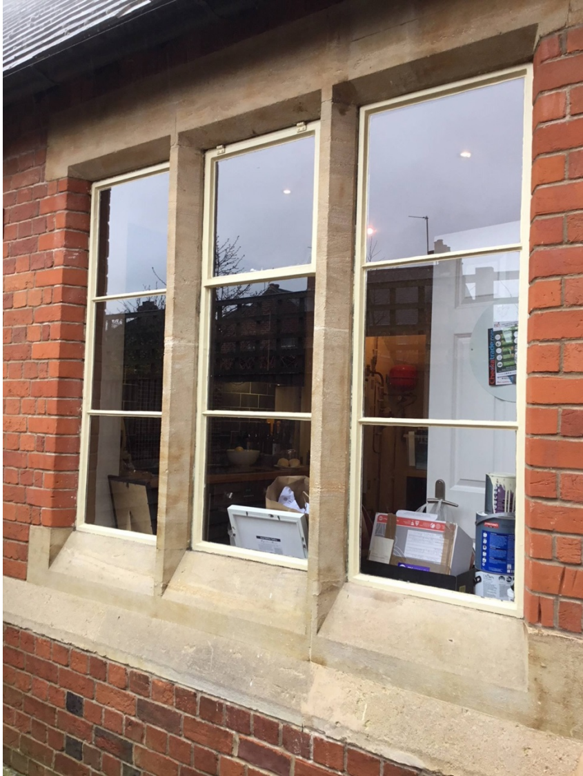
Windows to rear of property along eastern elevation
