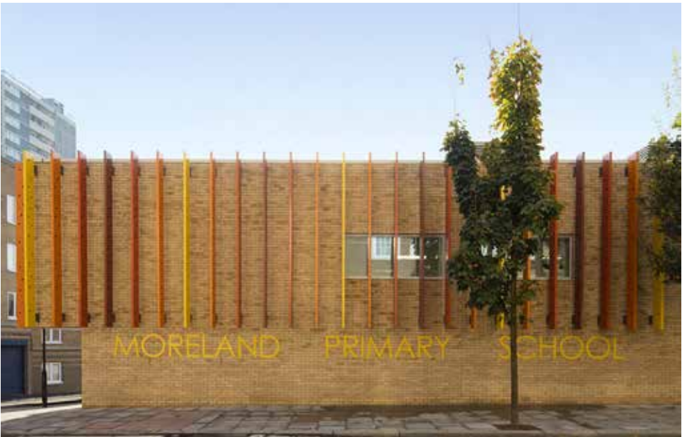
Example of coloured vertical shading fins and buff brick facade
