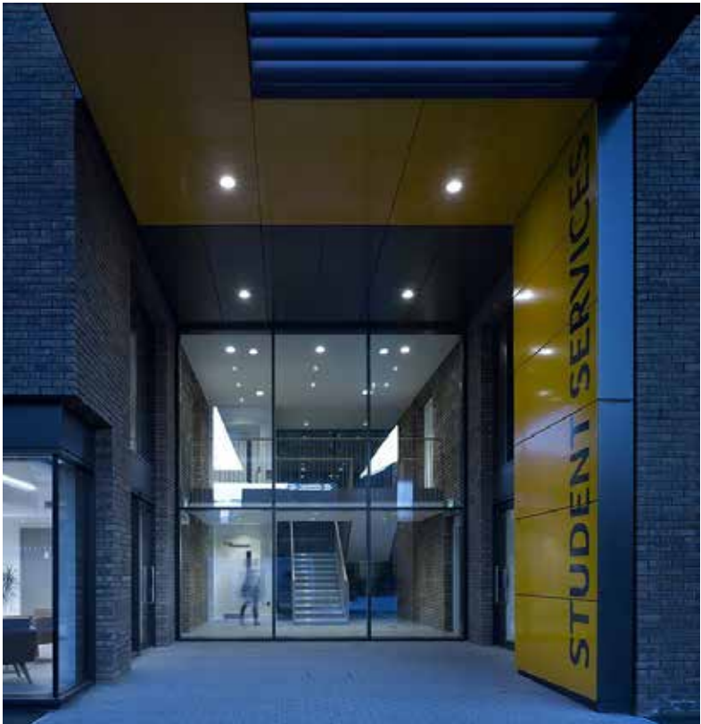
Example of coloured external wall panels signalling the main entrance
