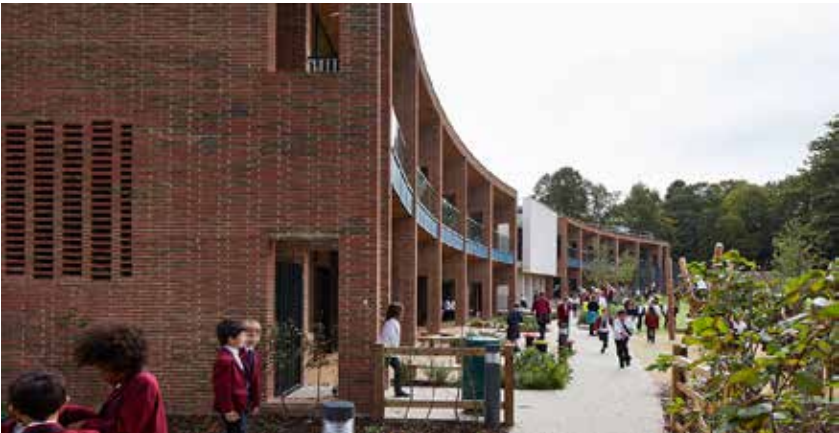
Example of external play area and curved facade
