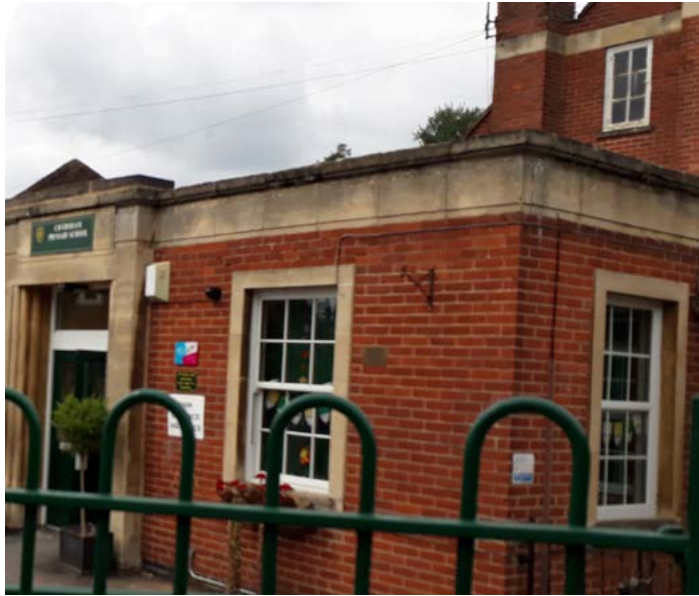
Brick on main school buildings
