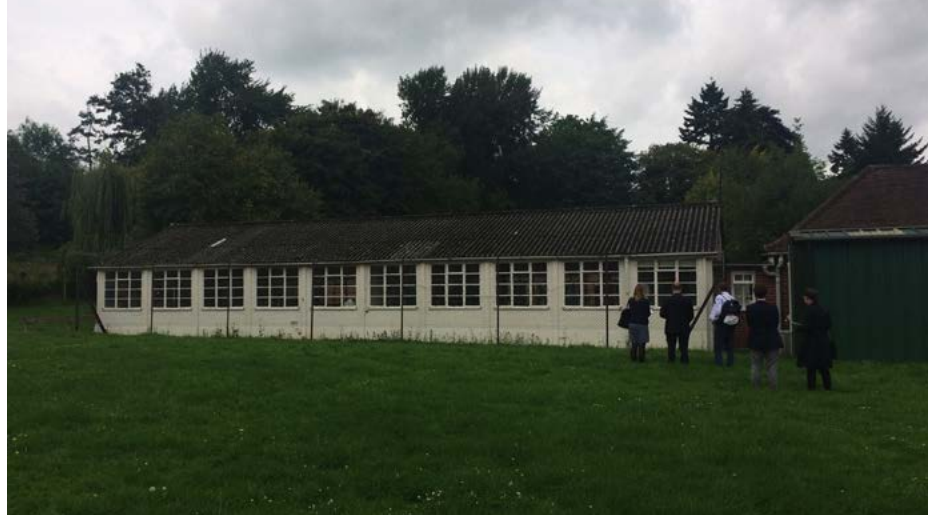
Existing View from South
