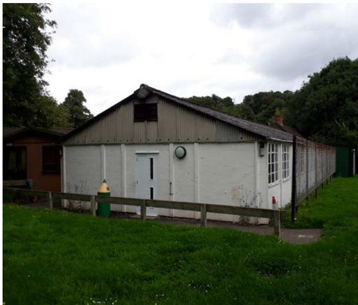
Building to be demolished
