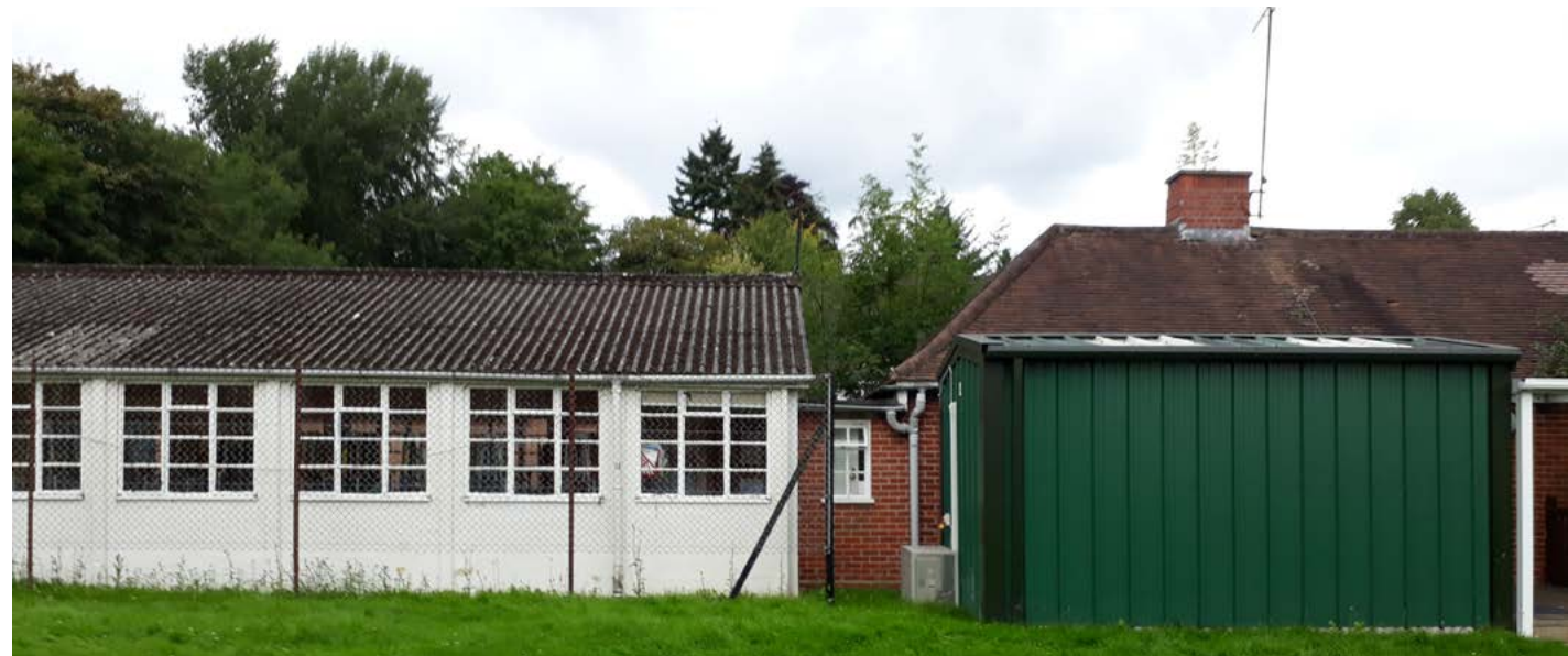
Building to be demolished adjacent to brick building
