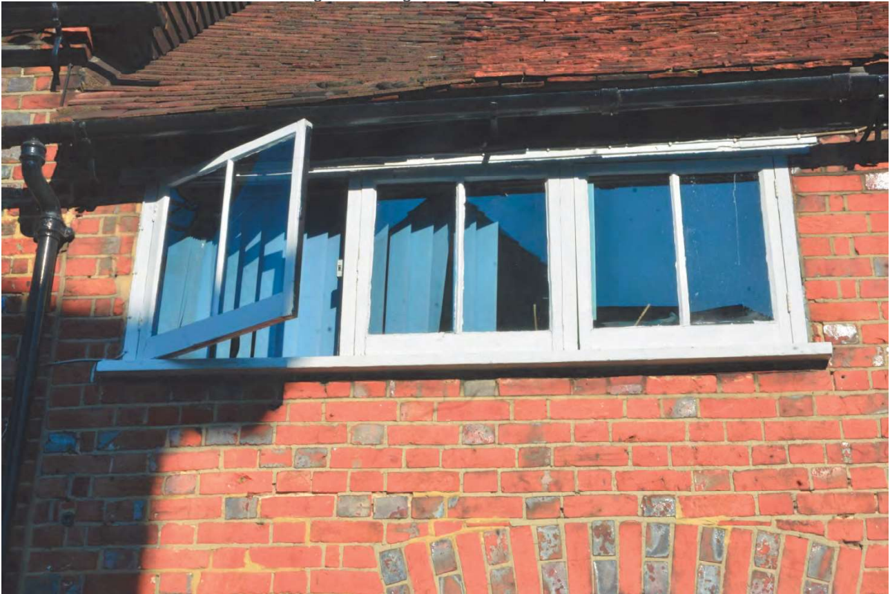
Plate 26: First floor central window
