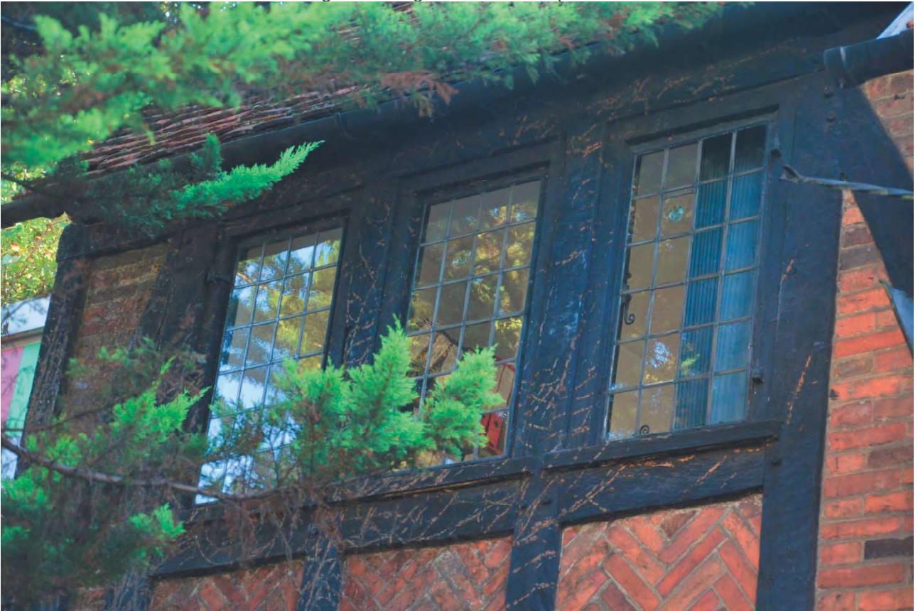
Plate 4: First floor southern window, no. 28
