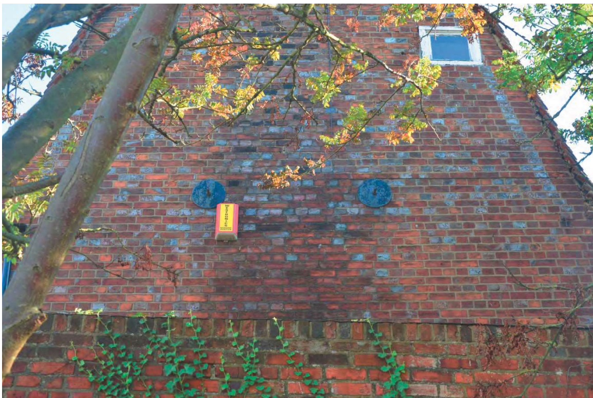
Plate 18: Detail of brickwork, north elevation
