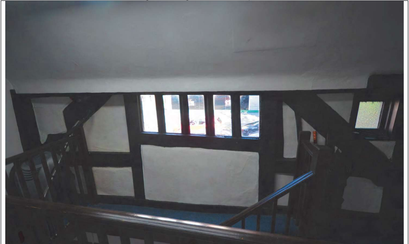
Plate 59: First Floor Room 1 Looking East
