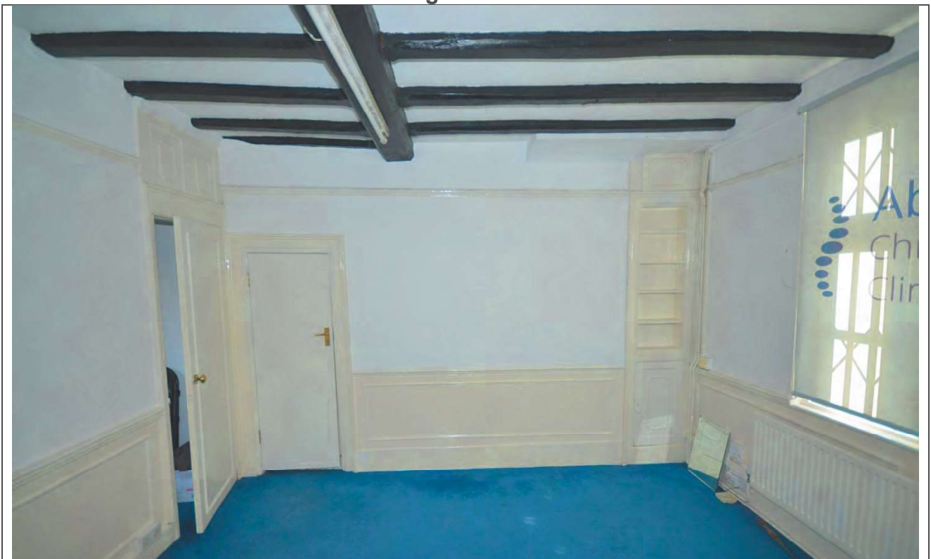
Plate 45: Ground Floor Room 5 Looking South
