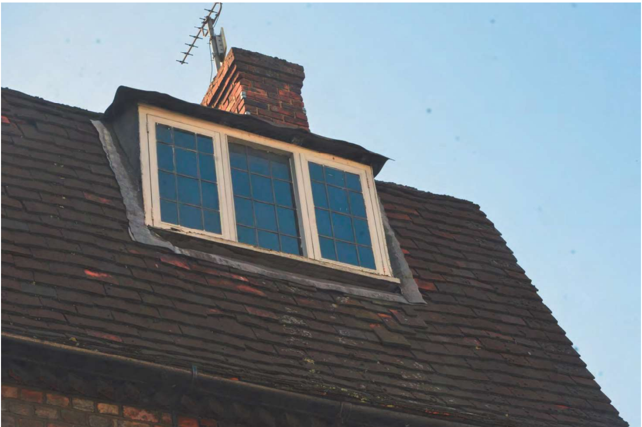
Plate 9: Dormer in mansard roof
