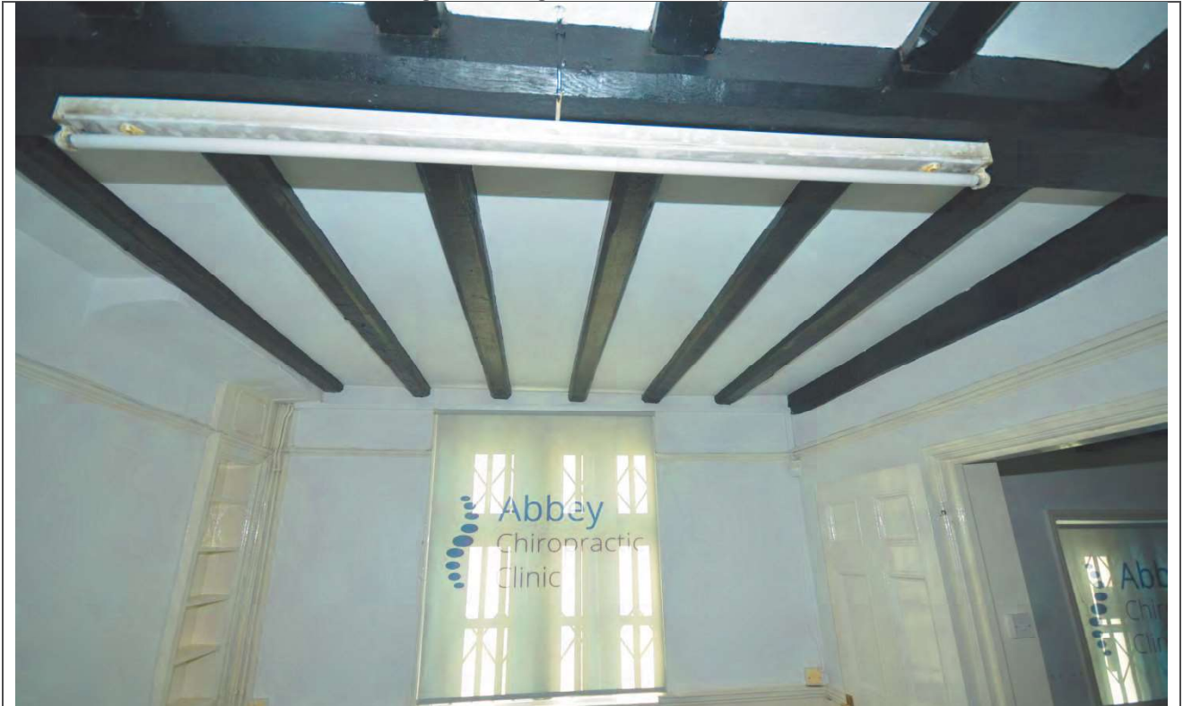
Plate 46: Ground Floor Room 5 Looking West
