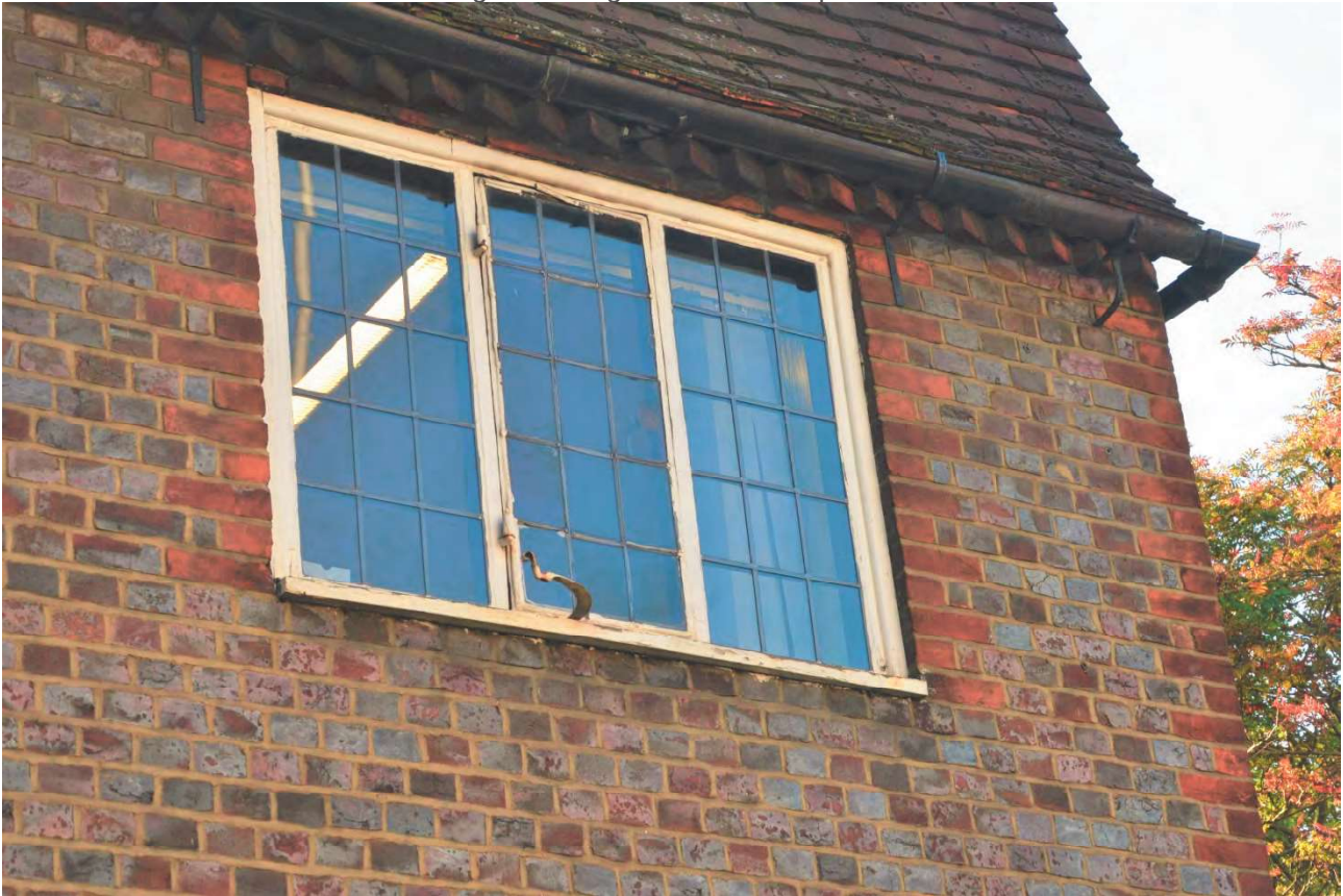
Plate 12: First floor iron-framed window
