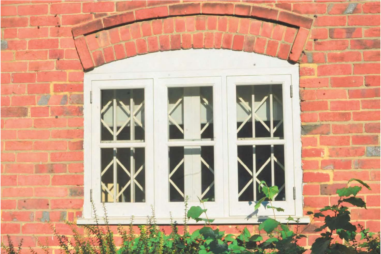
Plate 30: Ground floor south window
