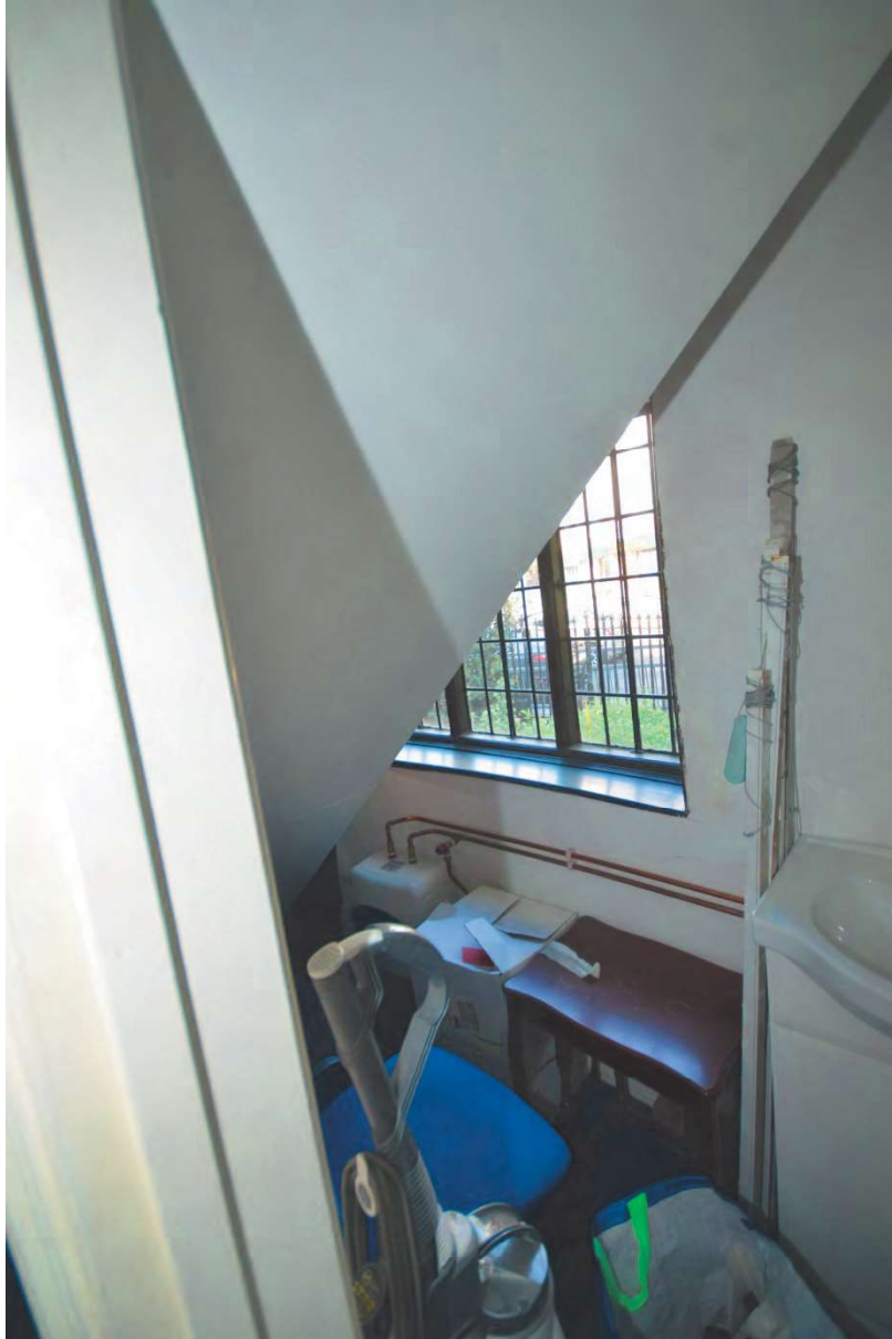
Plate 48: Ground Floor Room 5a Looking East
