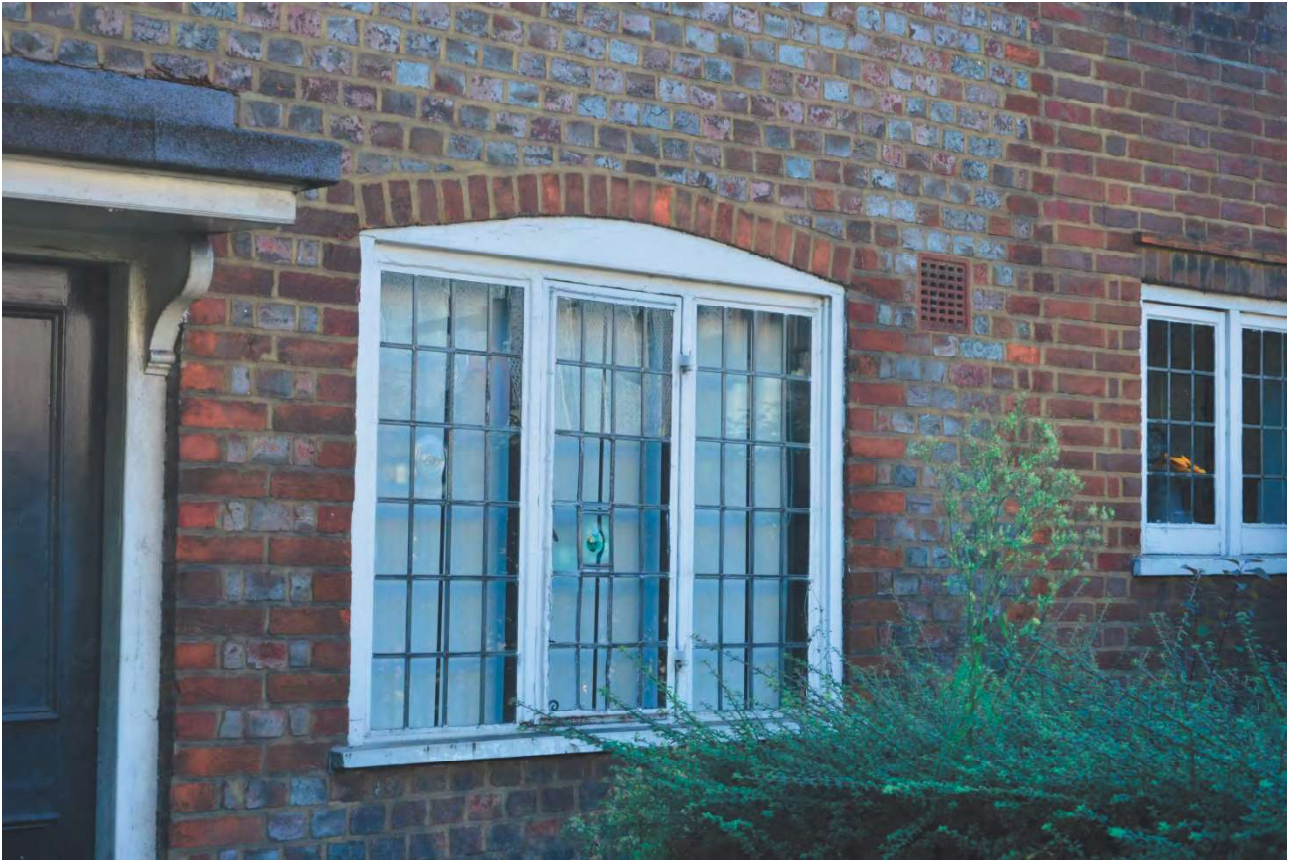
Plate 16: Ground floor iron-framed window
