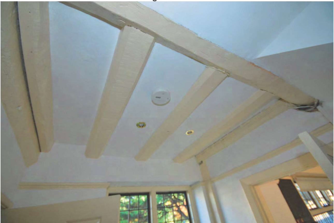
Plate 41: Detail of timbers in ceiling
