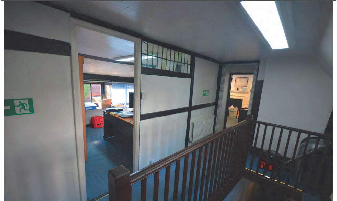
Plate 61: First Floor Room 1 Looking West
