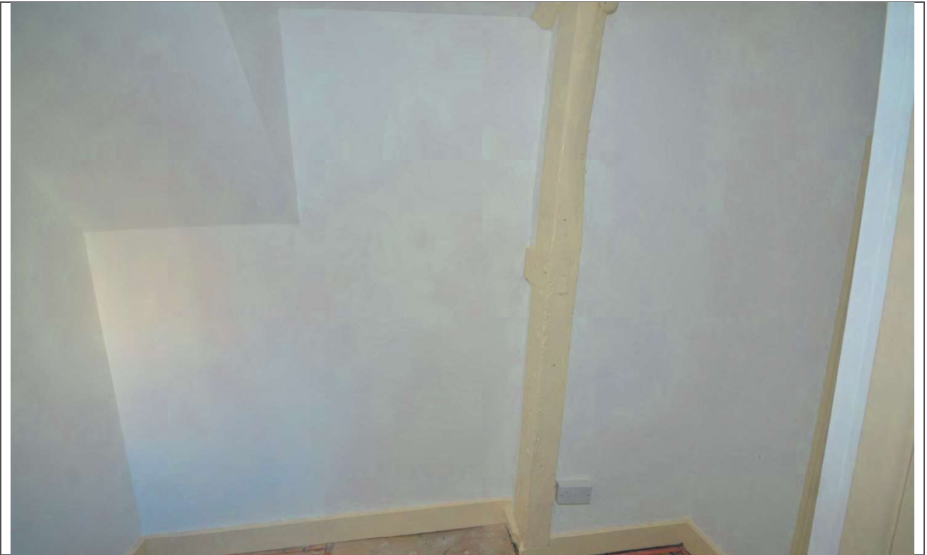
Plate 40: Ground Floor Room 3 Looking West
