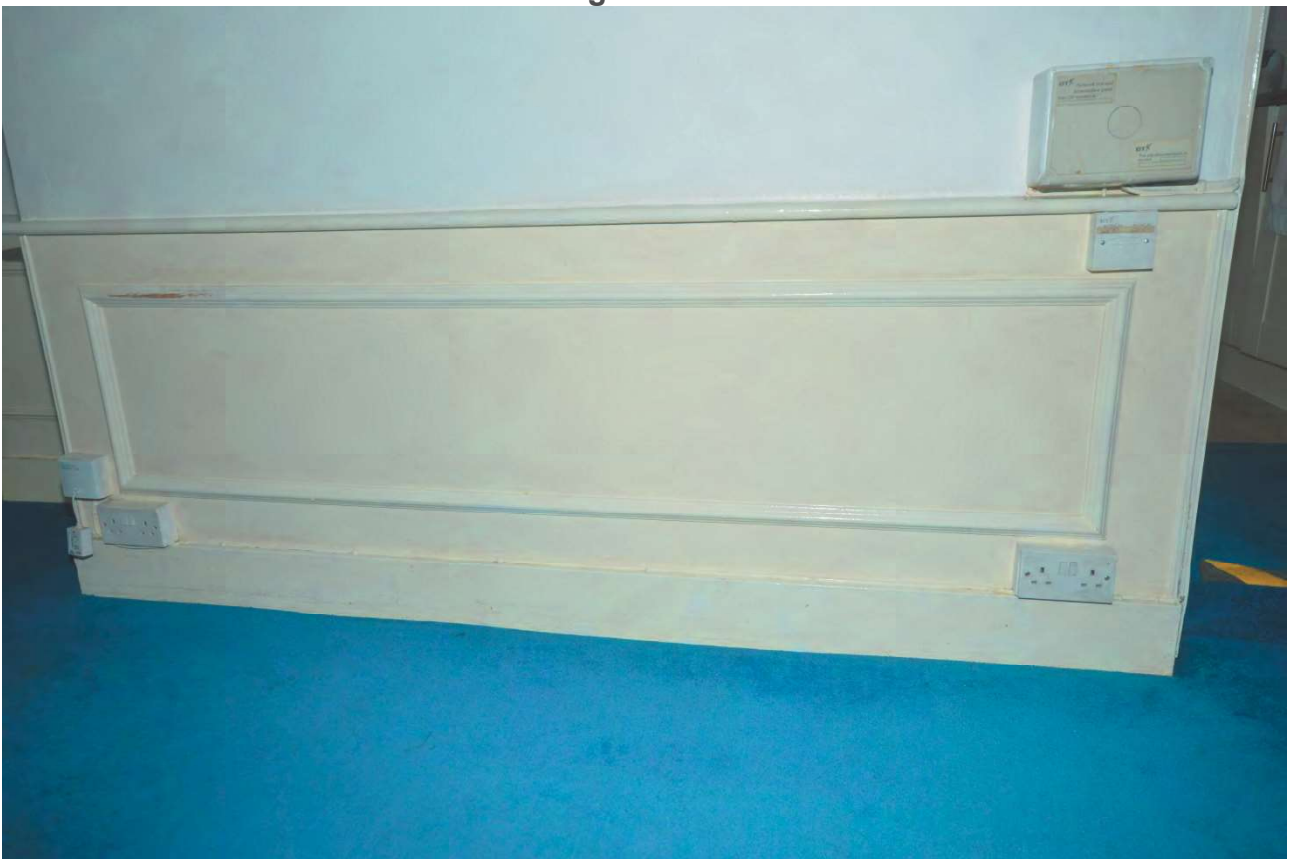
Plate 53: Detail of panelling across chimneybreast
