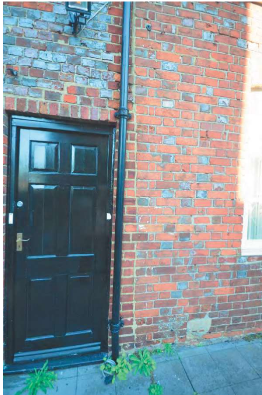
Plate 21: Clear distinction between brickwork in northern and central sections of the building
