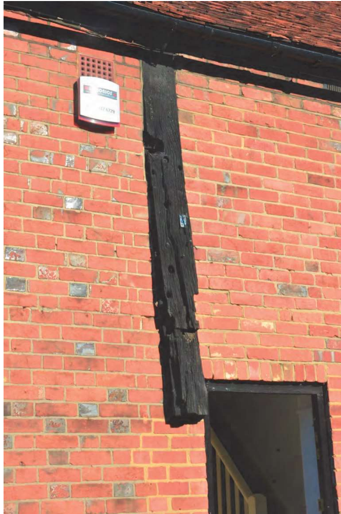
Plate 22: Timber dividing central and southern sections
