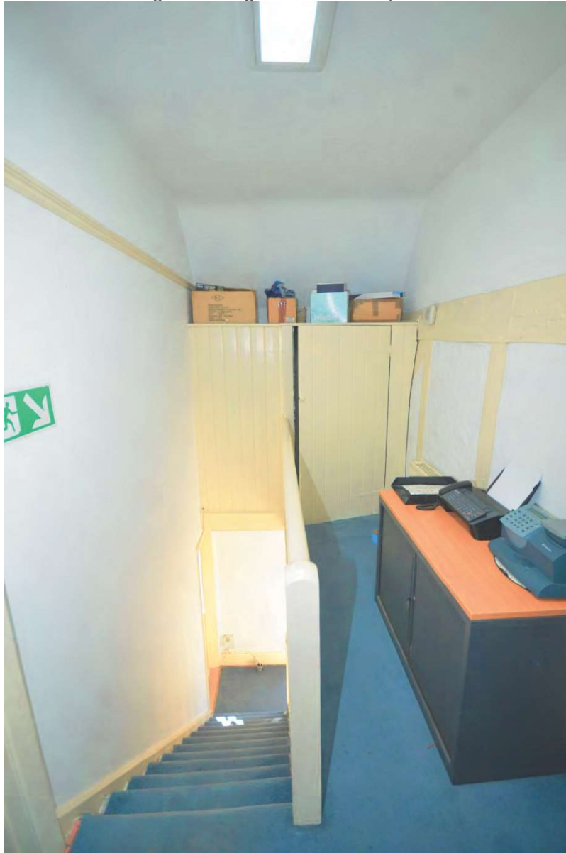
Plate 64: First Floor Room 2 Looking West
