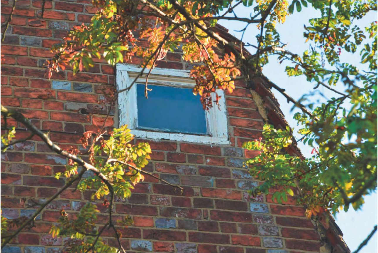
Plate 19: Detail of window, north elevation
