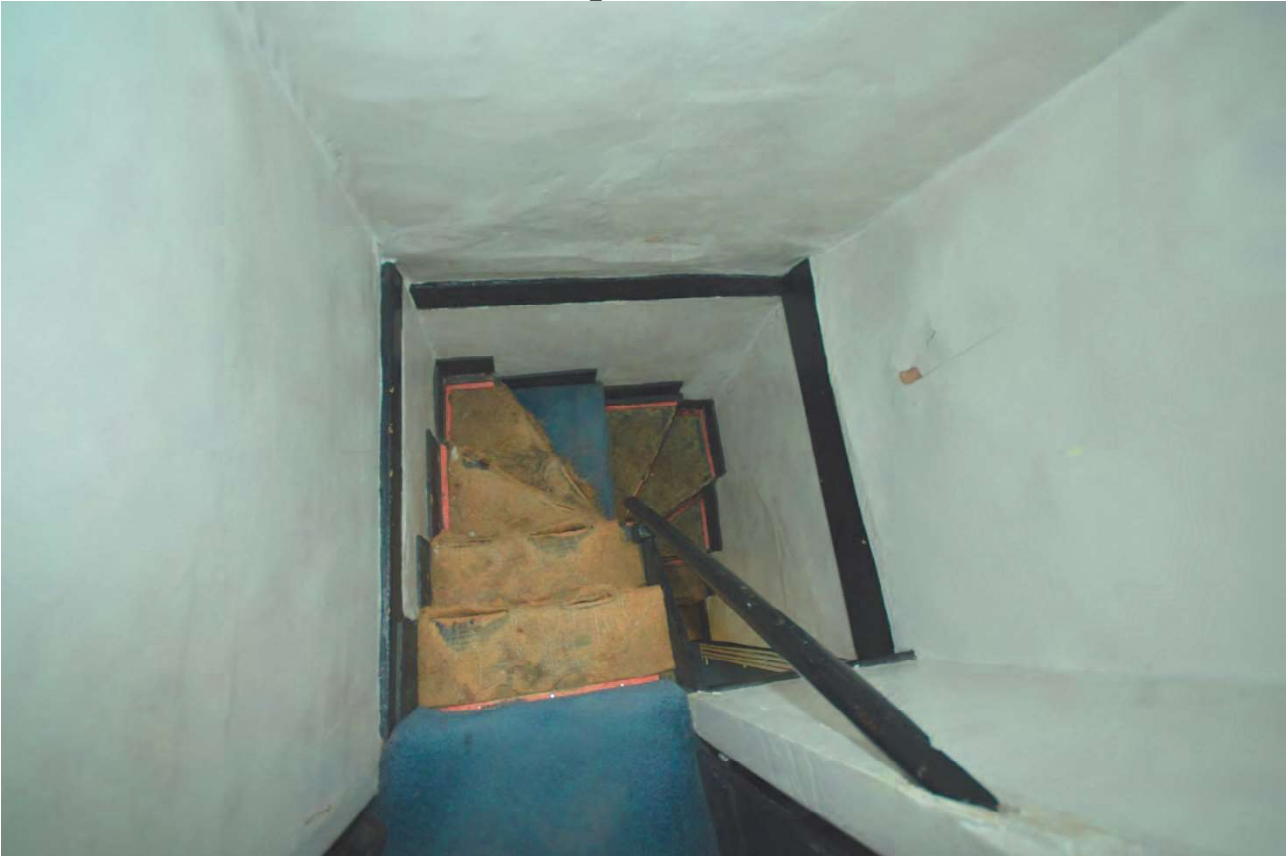
Plate 80: Staircase viewed from top
