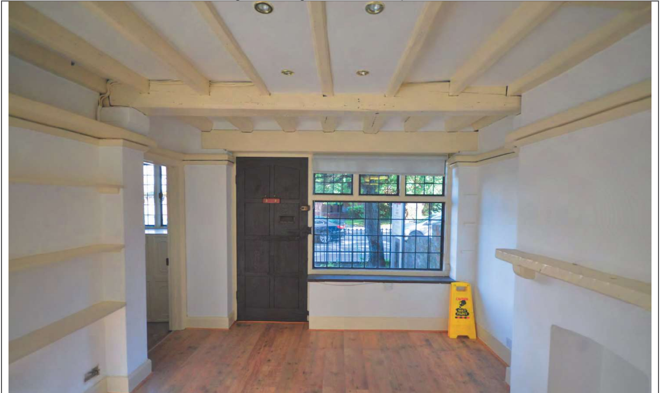
Plate 33: Ground Floor Room 2 Looking East
