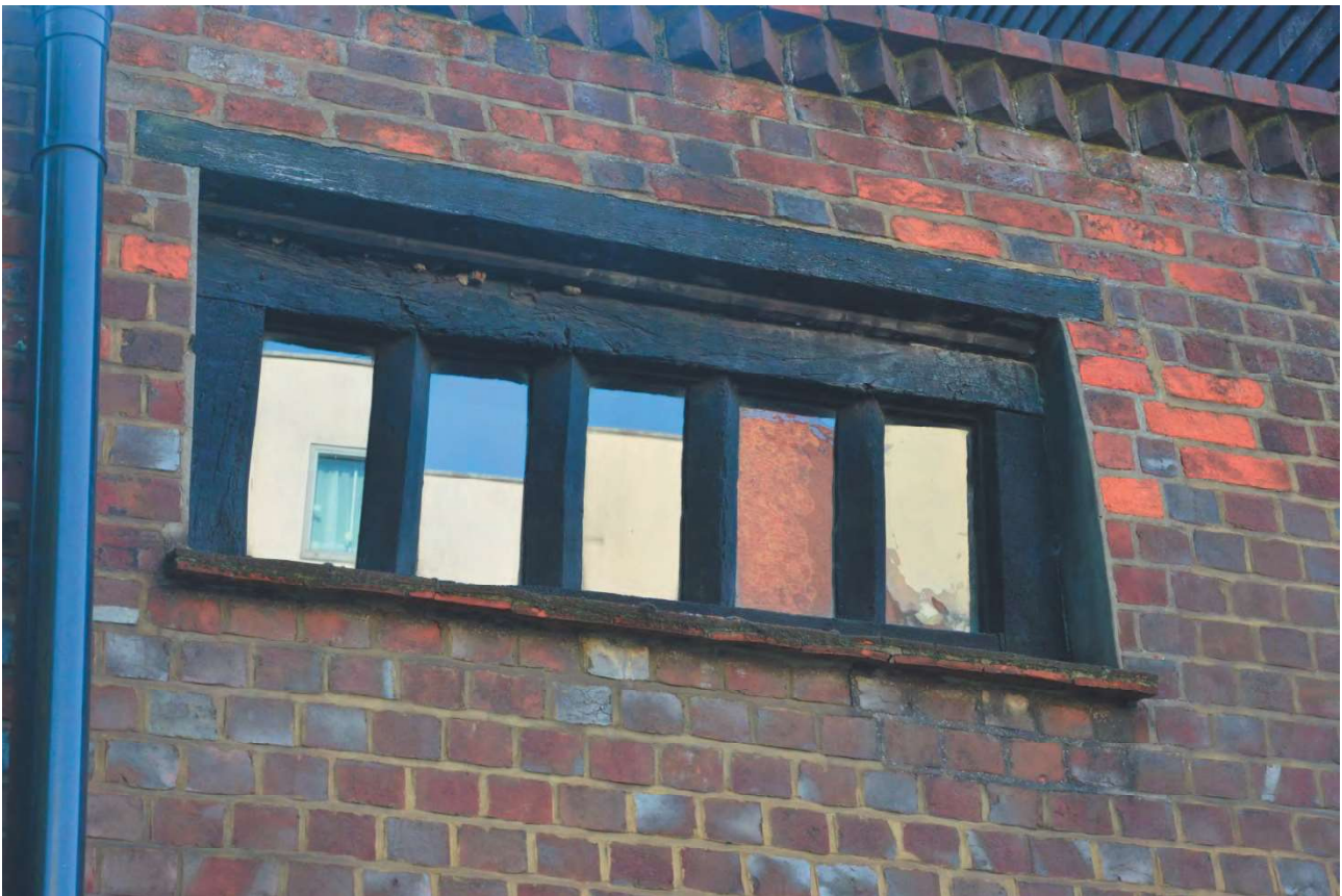
Plate 11: First floor timber mullioned window
