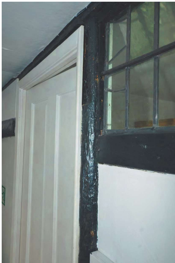
Plate 62: Detail of hand-sawn timber
