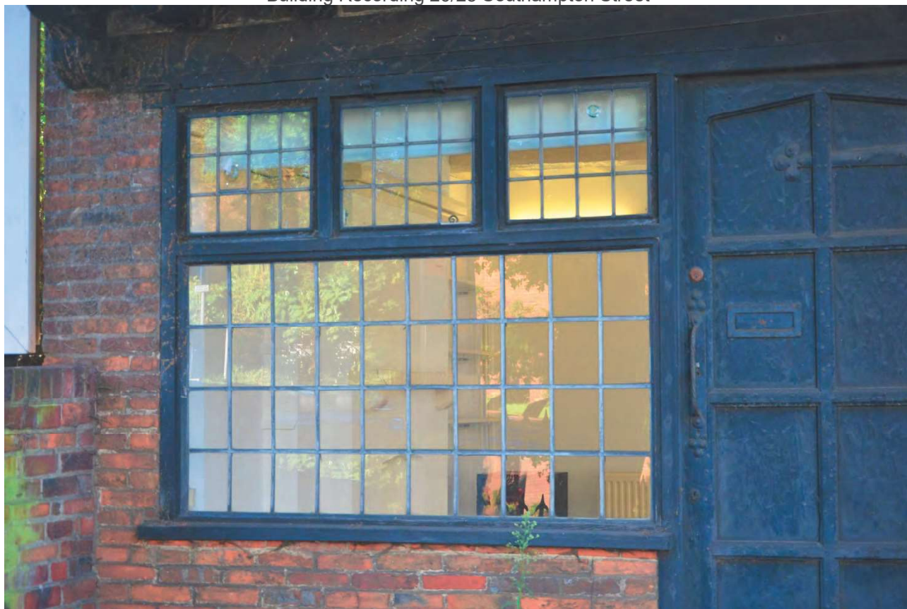
Plate 6: Ground floor southern window, no. 28
