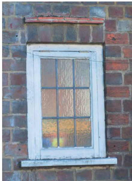
Plate 13: Ground floor top-hung casement
