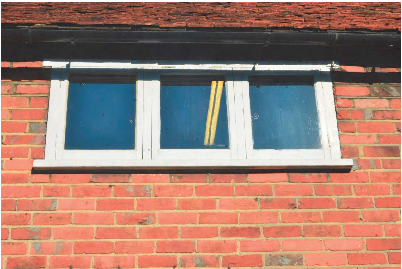
Plate 27: First floor south window
