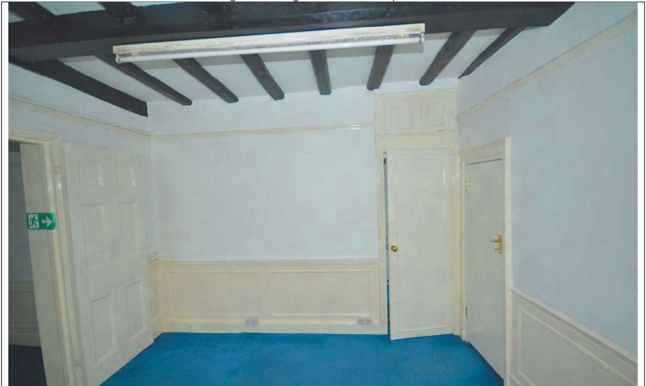
Plate 44: Ground Floor Room 5 Looking East
