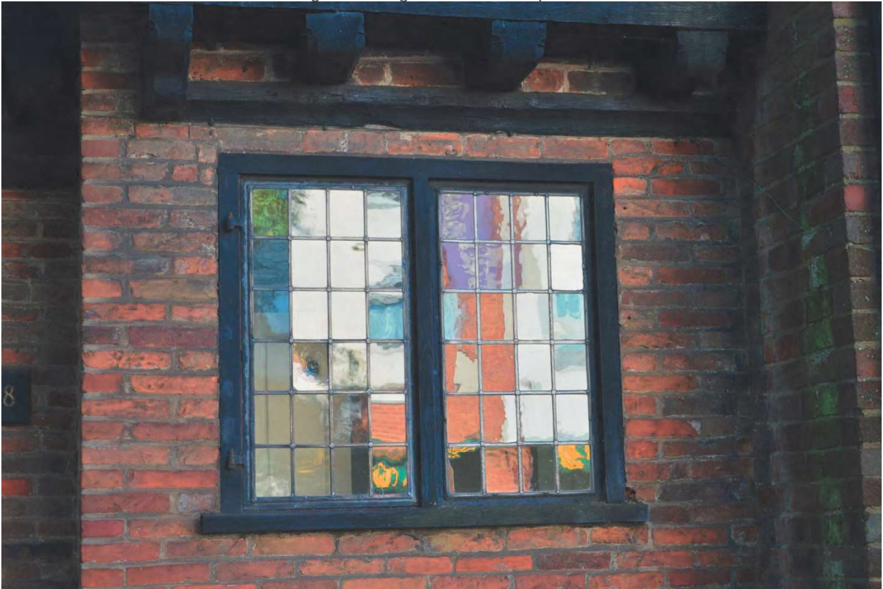
Plate 8: Ground floor north window with jetty beams, no. 28
