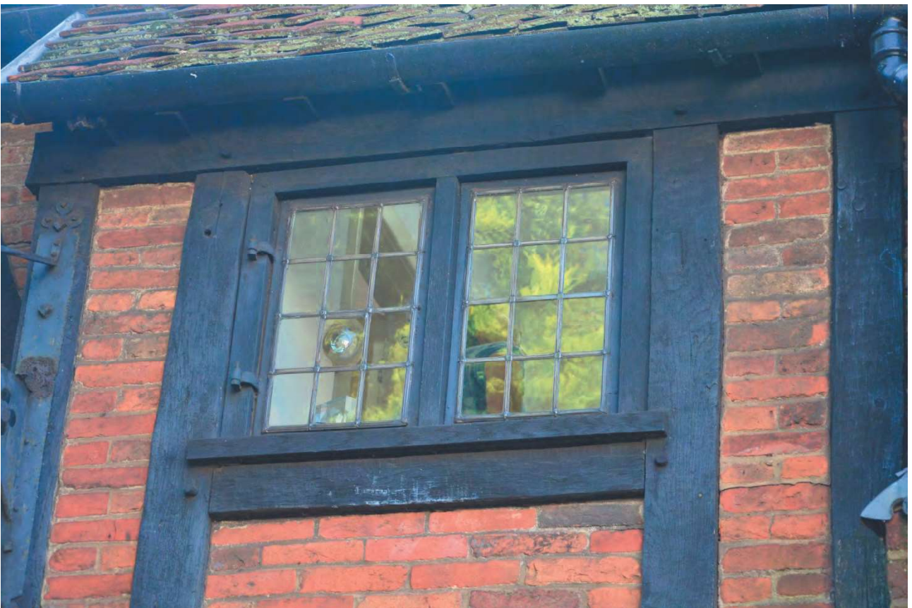
Plate 5: First floor northern window, no. 28
