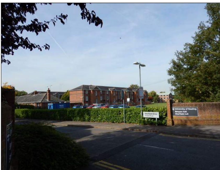
Figure 7: Public face of Pearson's Court from Northcourt Avenue – eastern & southern ranges.
