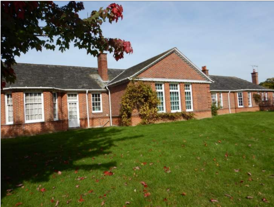
Figure 8: External elevation of southern range ('SETS' building).
