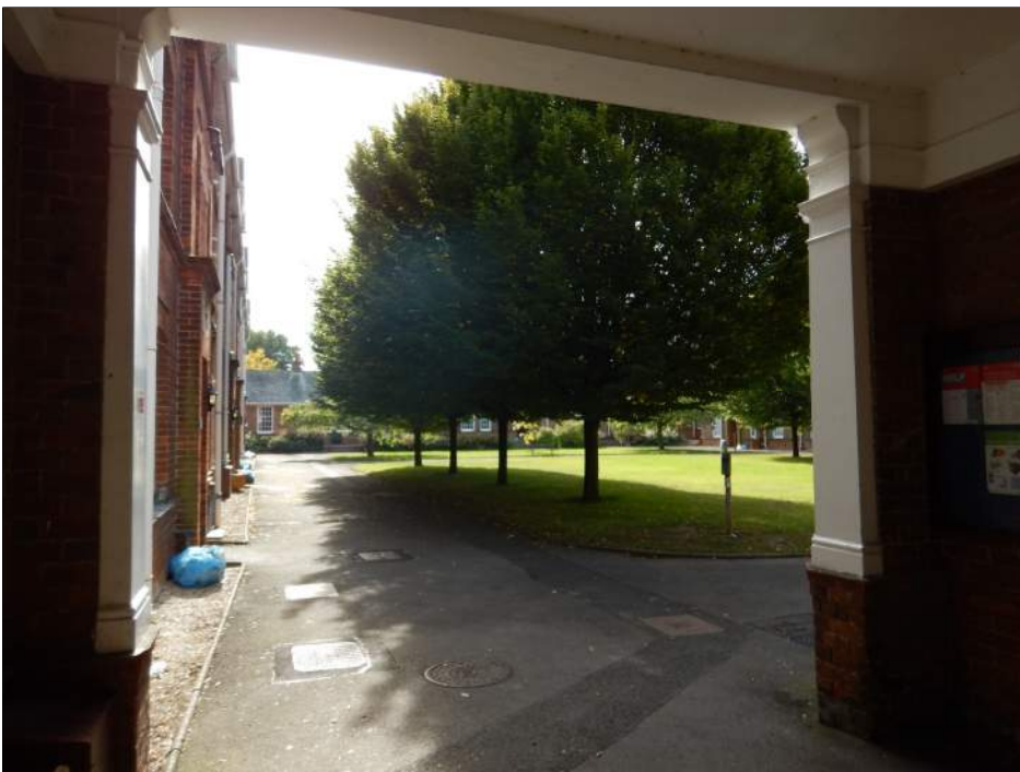
Figure 9: View from carriageway entrance on northern range into quadrangle with eastern range on left, southern range in background and western range on right.
