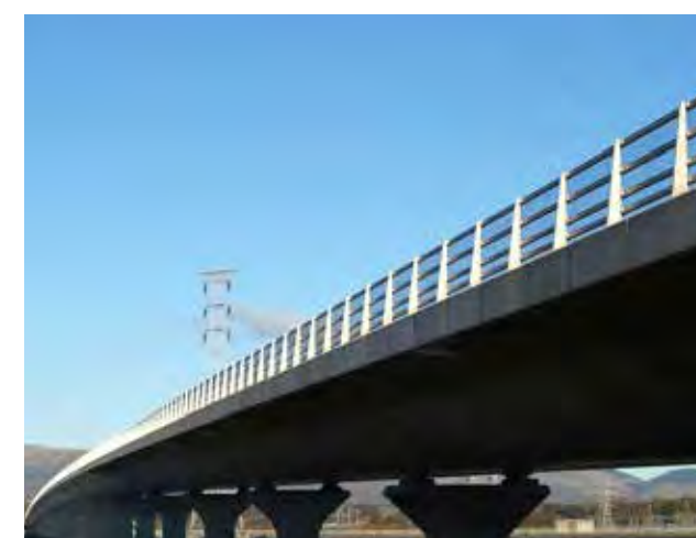
(Images: Stel Construction Info.)
