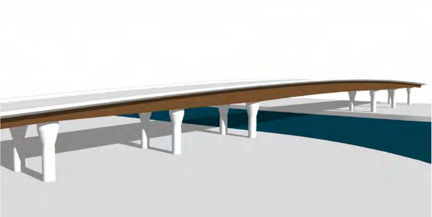
Deep, gently cambered girder to main river span tapering to the east and west.
