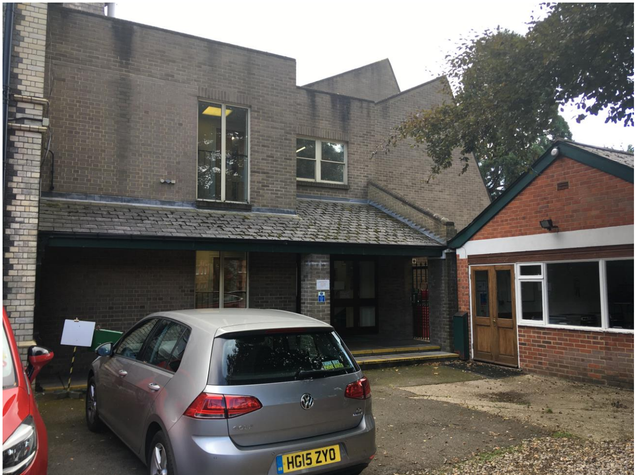
View of existing 1990's extension
