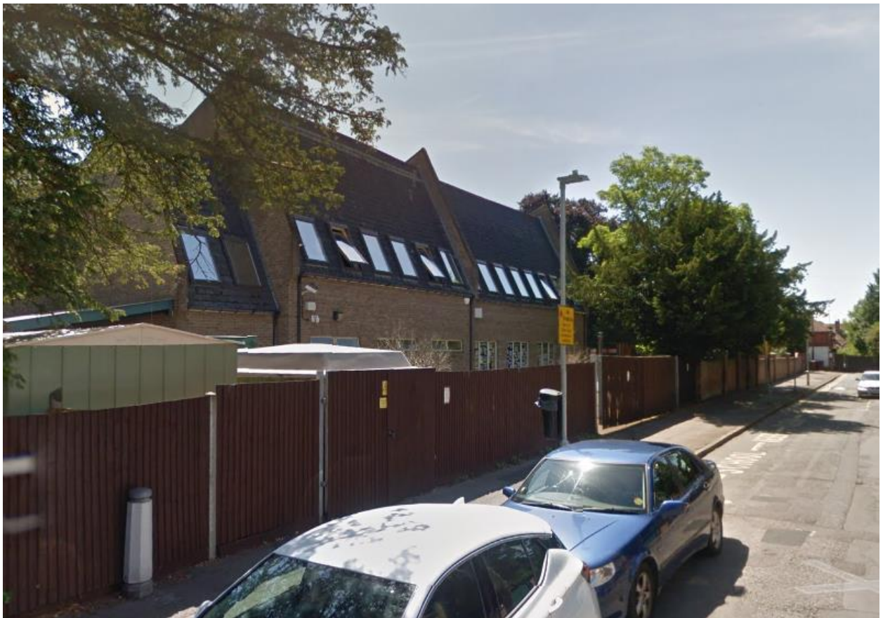
View of Existing Side Elevation from Vicarage Road
