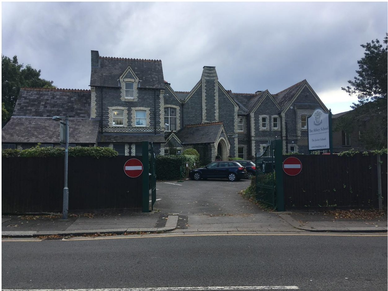
View of front of building from existing egress point
