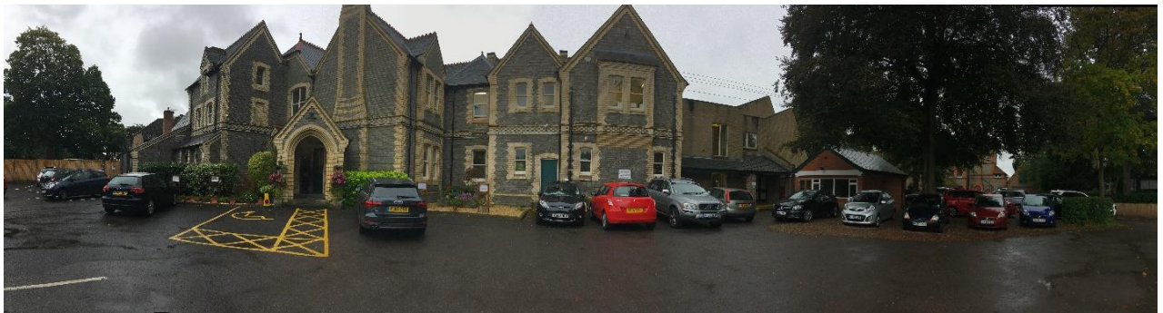
View of the front (north) elevation of the building
