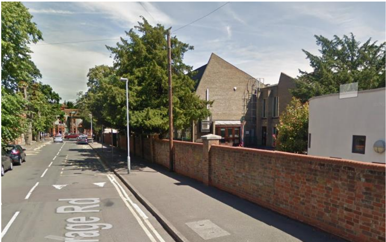
View of rear elevation from Vicarage Road
