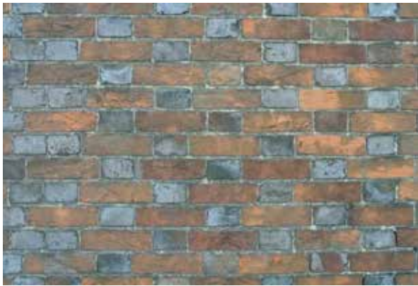
Simple decorative use of two bricks creating a Flemish bond with dark glazed headers and soft red stretchers along Watlington Street
