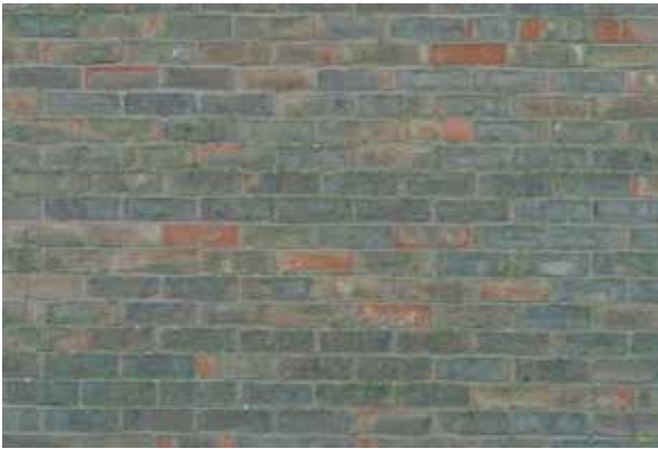
A naturally weathered and stained red brick wall within the Endon Street Conservation Area
