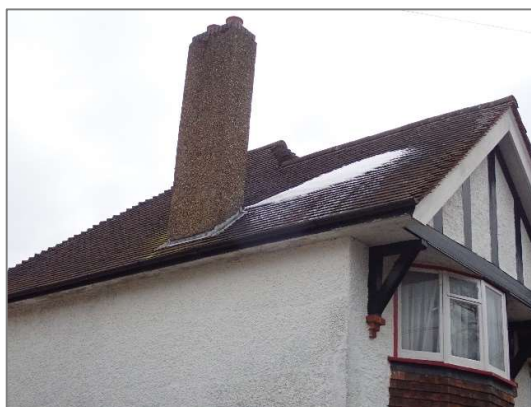
Photo 2 – Tiles to side roof pitch in good condition
