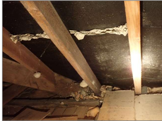
Photo 12 – Newspaper packed behind roofing felt
