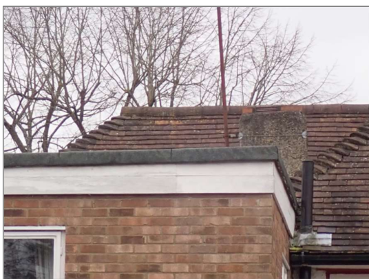
Photo 3 – Rear of house showing flat roof extension and tiles to main roof
