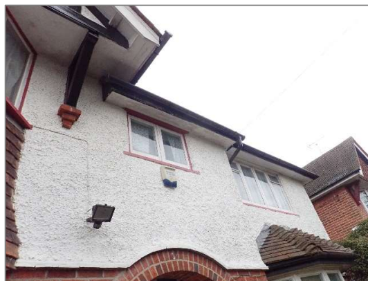
Photo 6 – Soffits to front elevation
