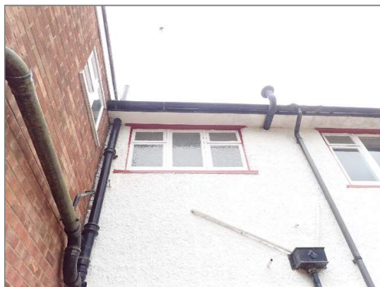
Photo 5 – Soffit to rear elevation
