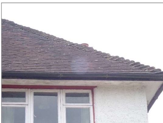
Photo 1 – Roof tiles to rear roof pitch in good condition
