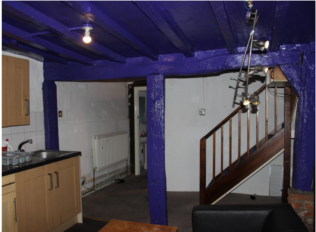
Figure 5 No. 38, front room with exposed ceiling joists.
