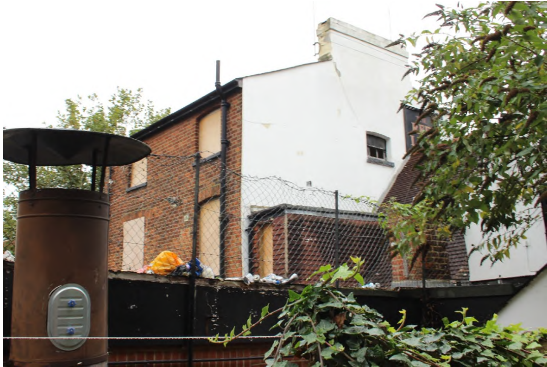
Figure 3 Rear elevation above the single storey extension with the rendered south elevation to the right.
