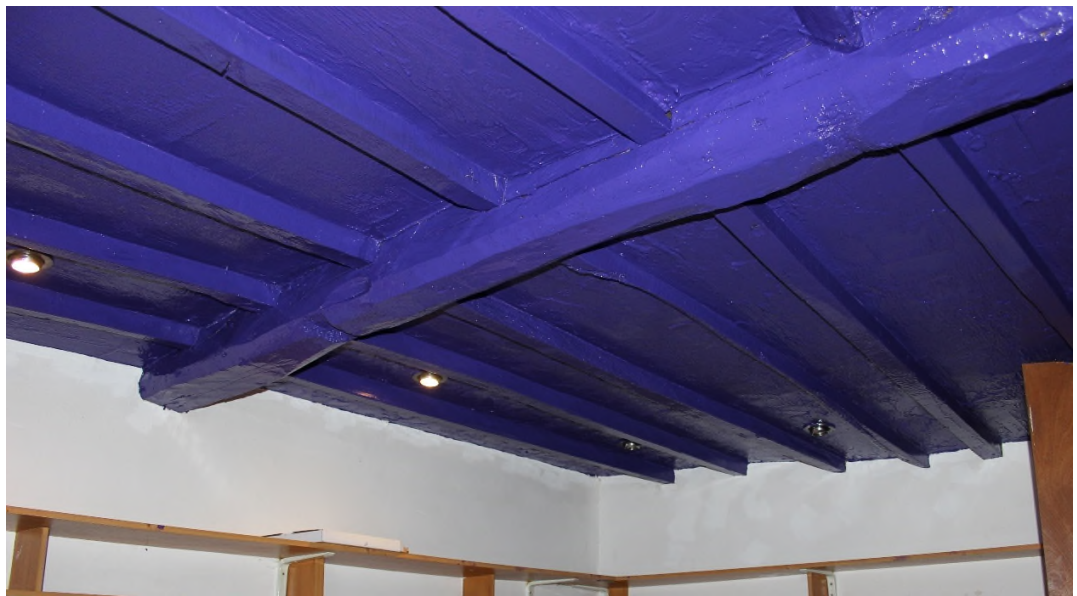
Figure 6 Ceiling beams to the first floor bedroom within the single bay of No. 38.
