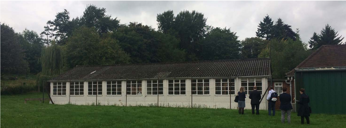
1- Block to be demolished, view from the south
