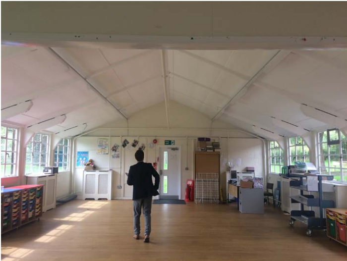
2- Interior of block to be demolished
