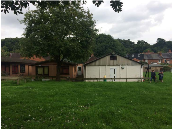
3- Block to be demolished, view from the west
