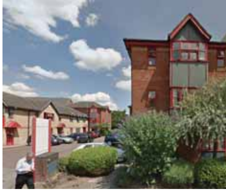
3 Storey Windsor Court - adjacent to the site
