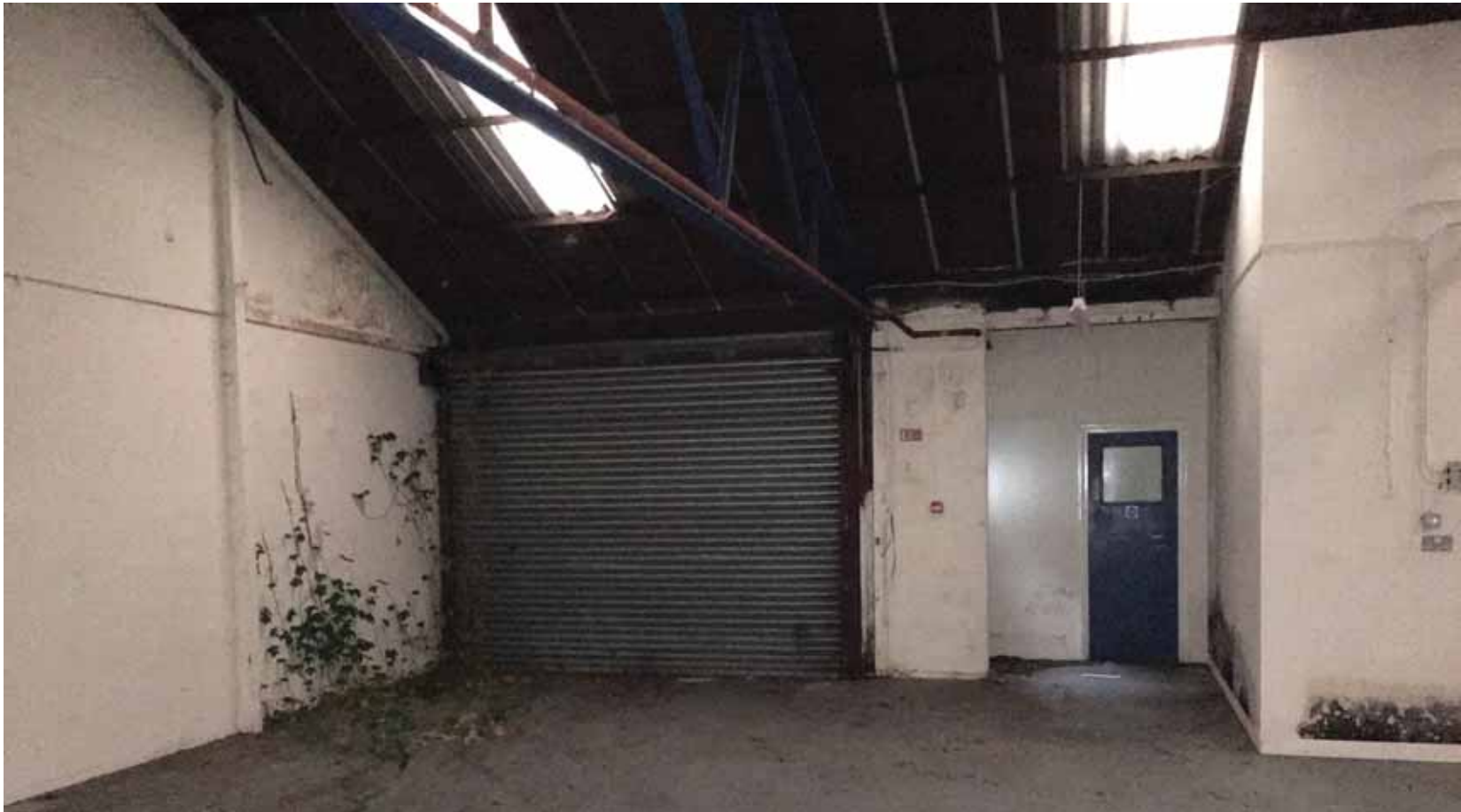
INTERNAL: EXISTING SITE VIEW
