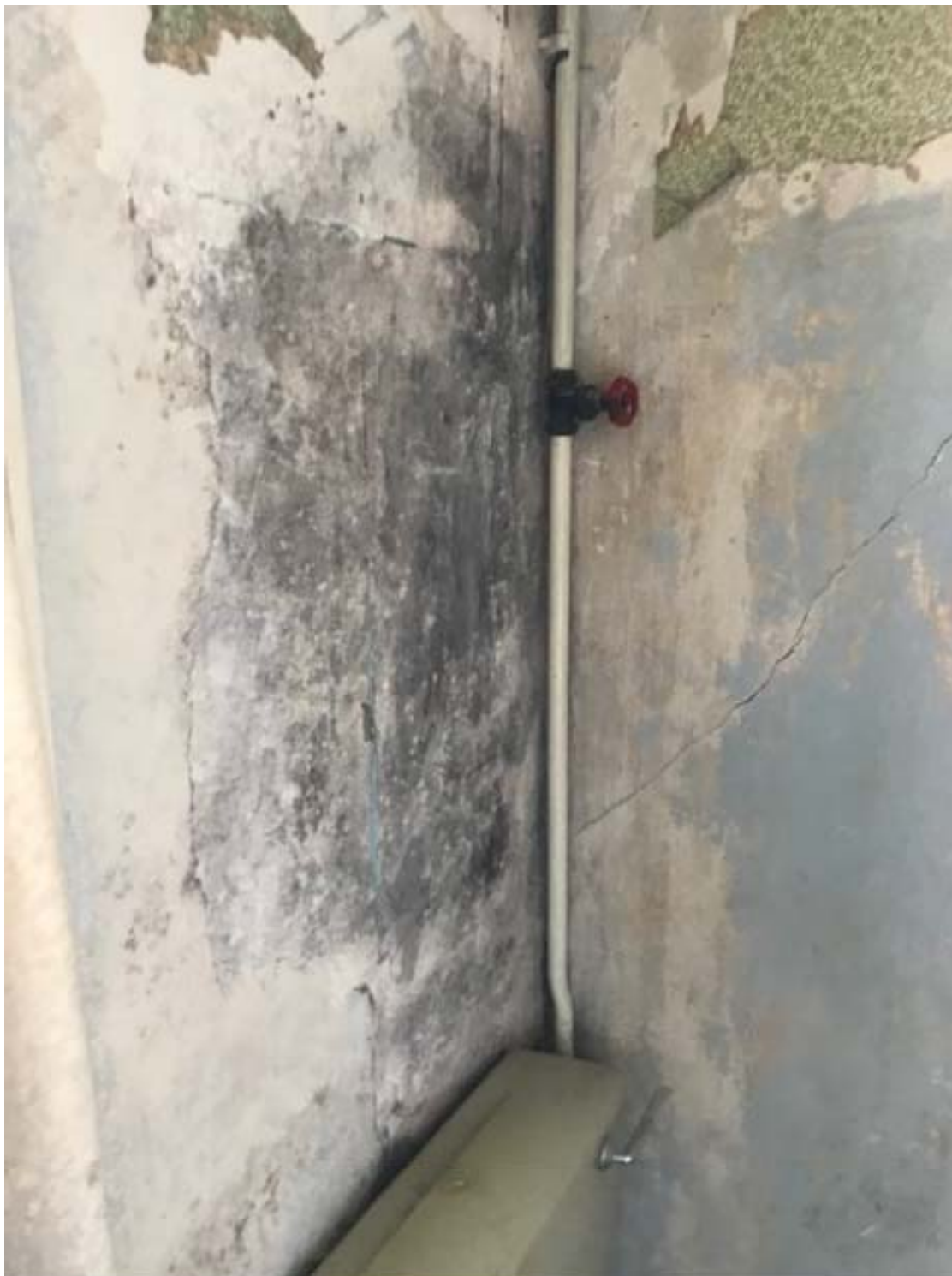
Fig C – Wall to bathroom behind WC
