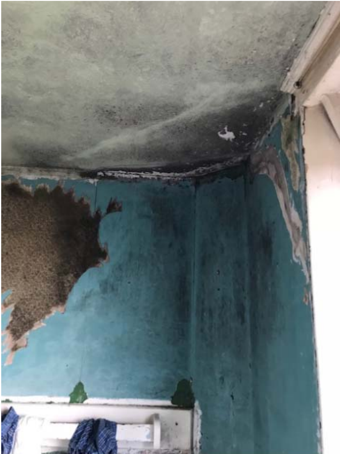
Fig D - Corner of bathroom
