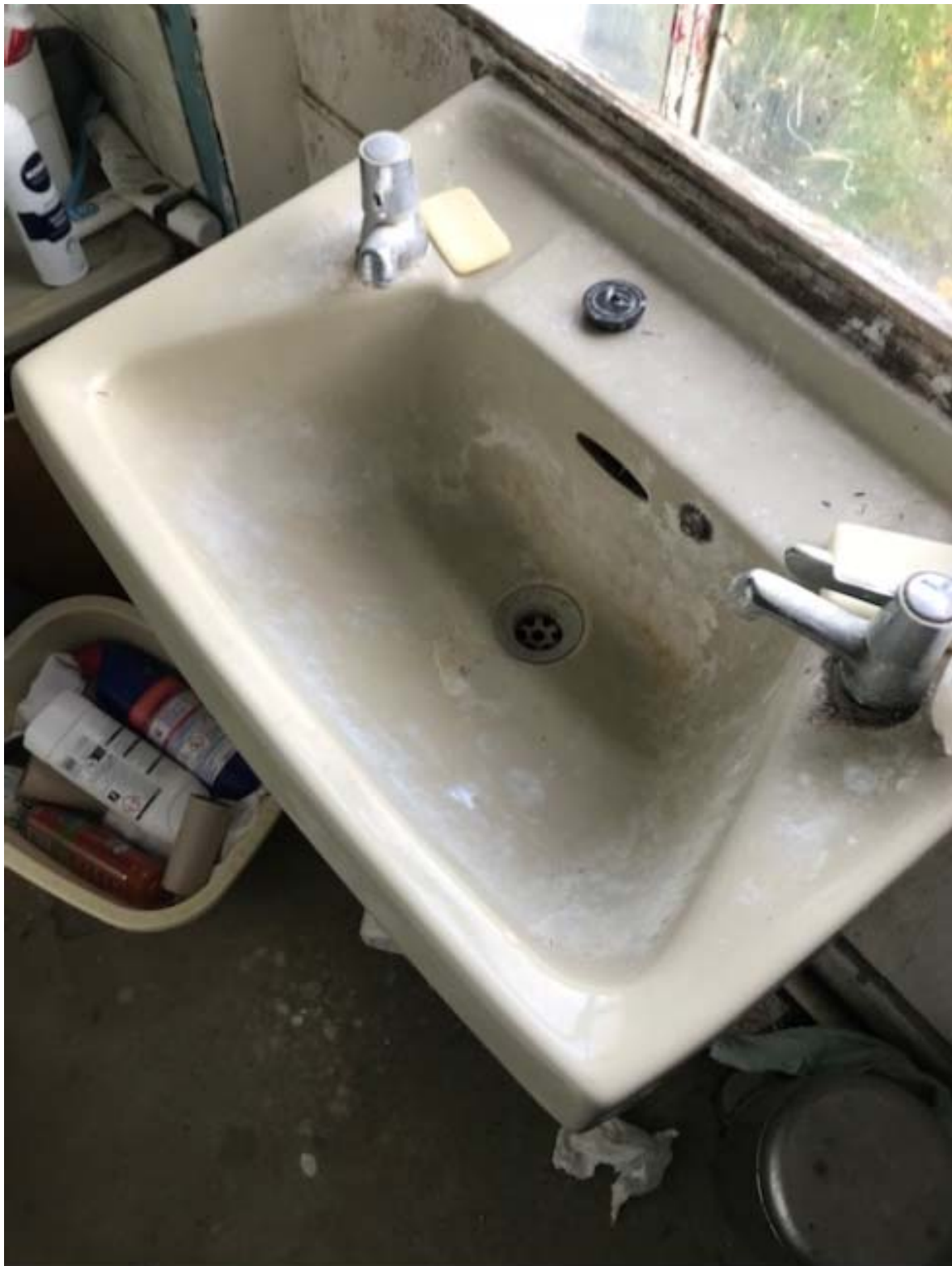
Fig B - Existing sink in front of Wi-Ex02
