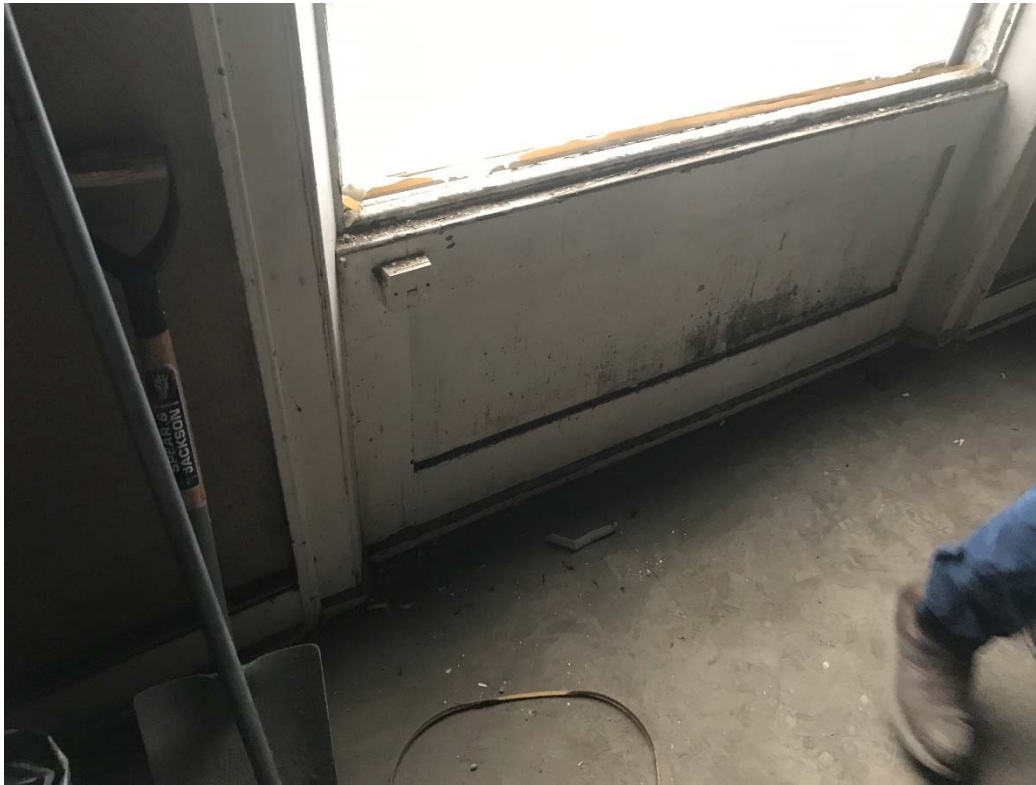
Fig 7 - Panelling beneath windows
