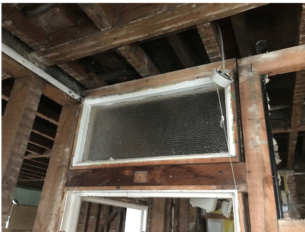
Fig 6 - Retained fan light over existing door
