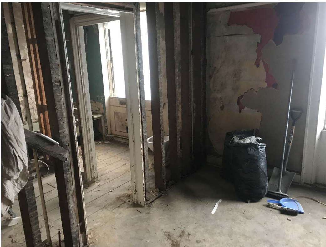
Fig 4 – Studwork removed from studwork wall between rooms
