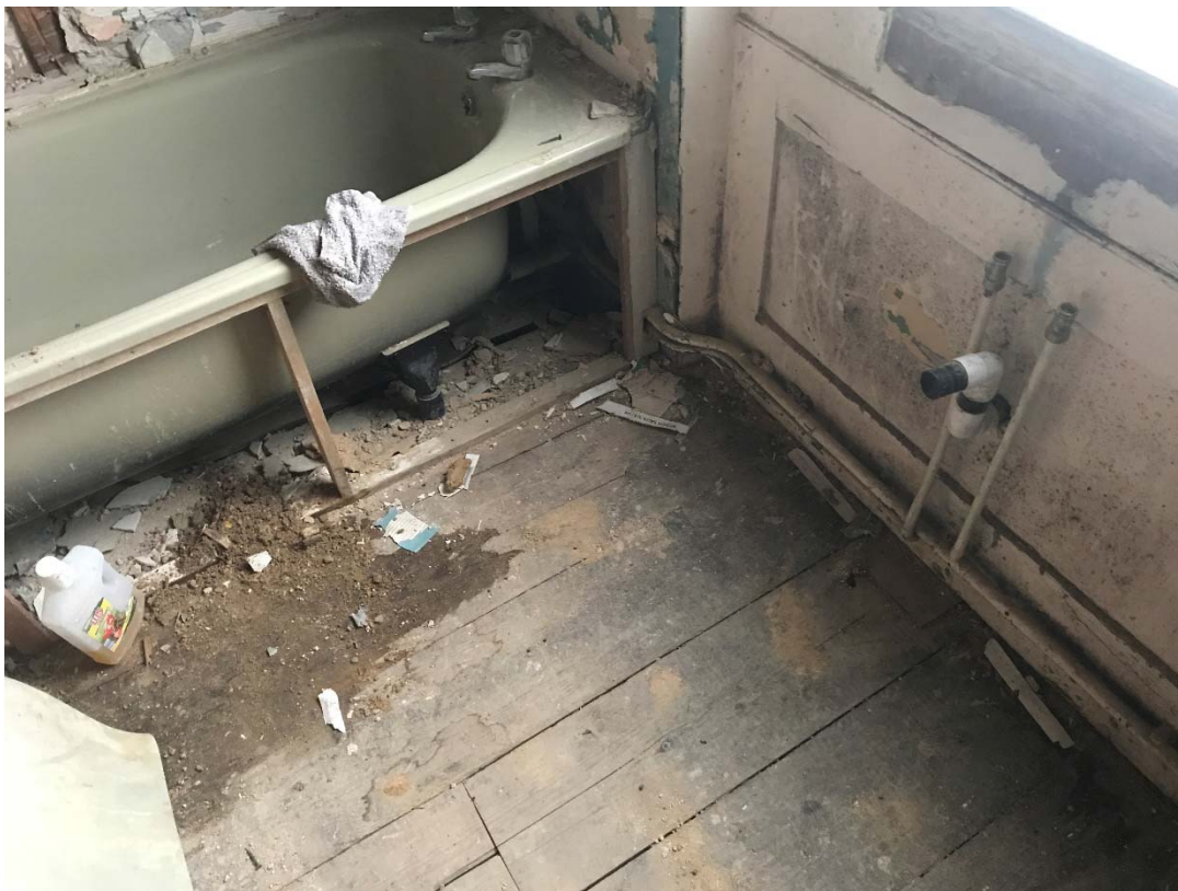
Fig 10 - Removed sink and bathroom furniture
