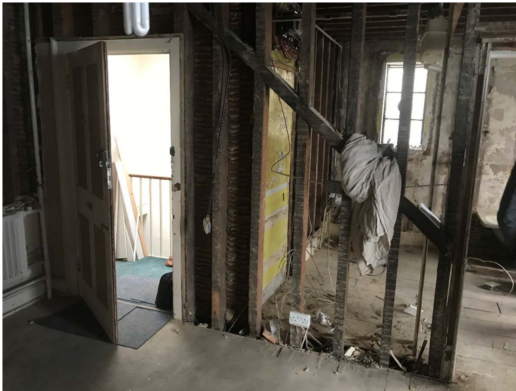
Fig 1 - Front door, studwork wall that separates living and kitchen area
