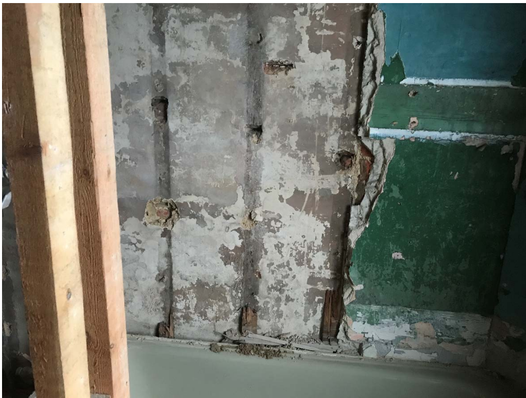
Fig 8 - Softwood drylining to bathroom, removed
