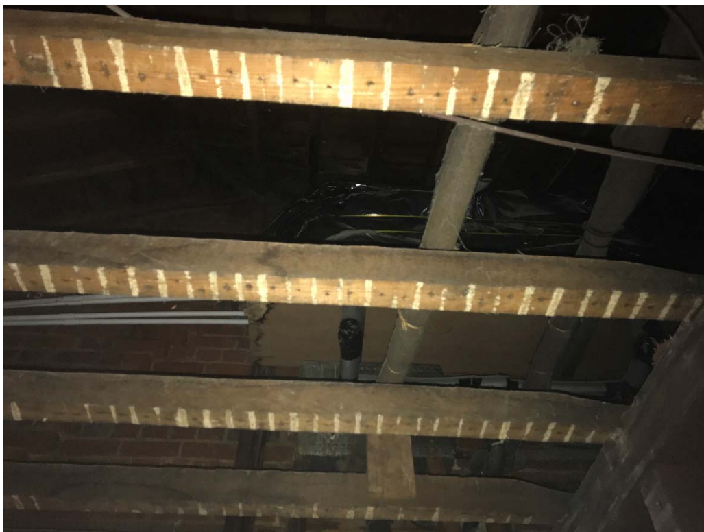
Fig 5 - Removal Lath and Plaster ceiling to expose joist
